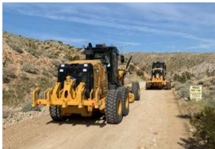
Motor graders performing routine grading along the CRA
