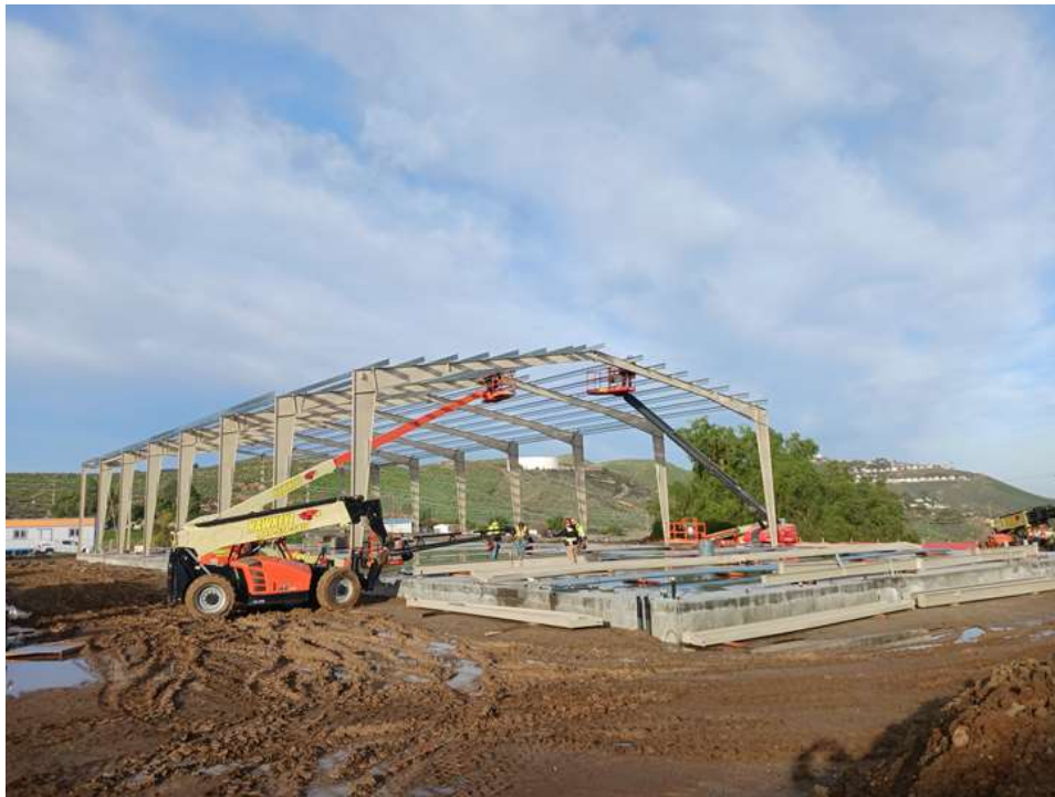
PCCP Rehabilitation Valve Storage Building —Erection of steel framing
