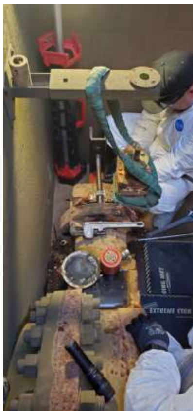
Staff replacing an influent valve gearbox at the Skinner plant
