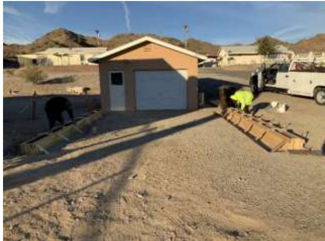
Staff tying rebar (left) and constructing concrete formwork (right) at Desert housing structures
