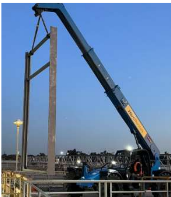
Weymouth Basins 5-8 and Filter Building No. 2 Rehabilitation—Installing gate guide
