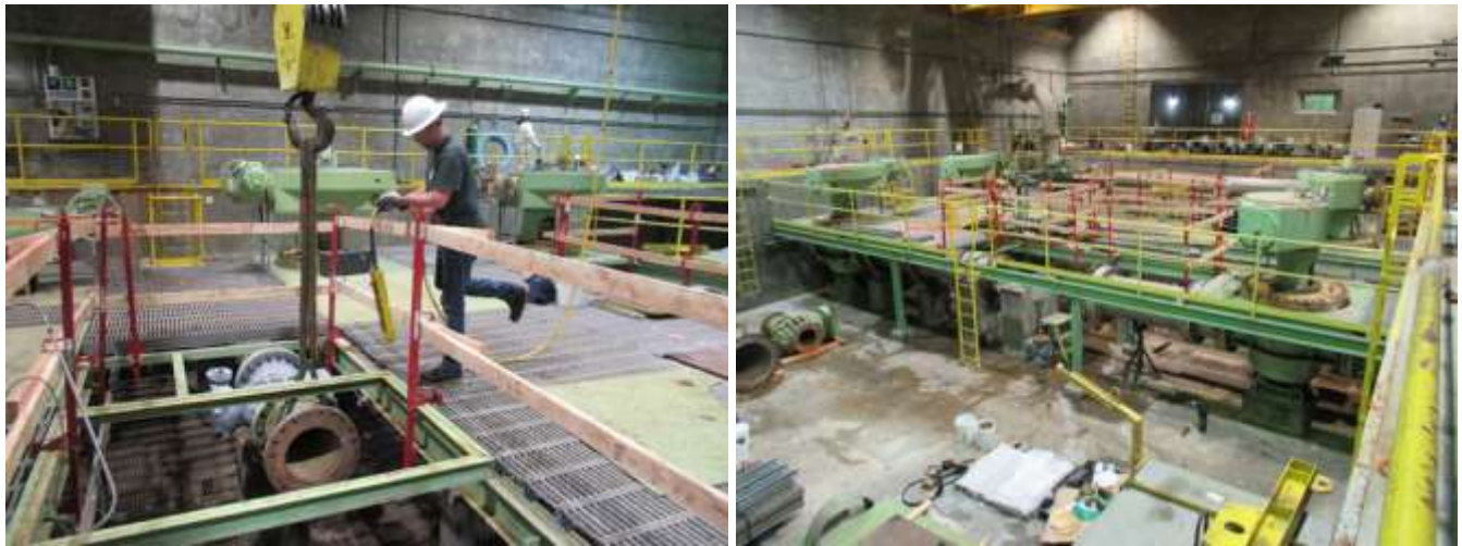
Staff replacing valves at Oak Street PCS
