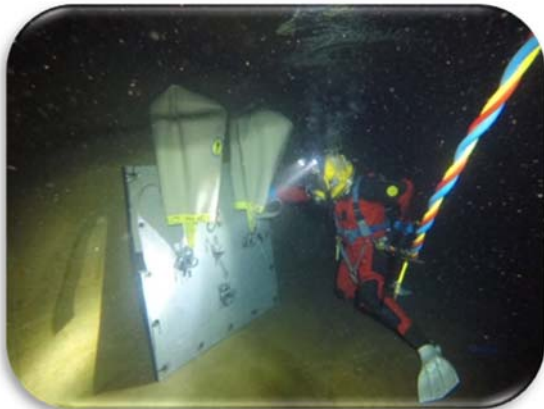
Diver positioning isolation plate at Diemer plant
