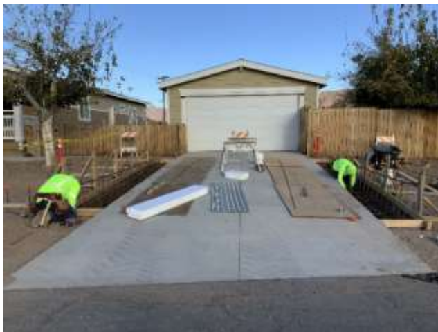
Staff tying rebar (left) and constructing concrete formwork (right) at Desert housing structures
