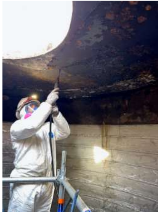
Staff removing aged coating inside a chamber at Red Mountain HEP
