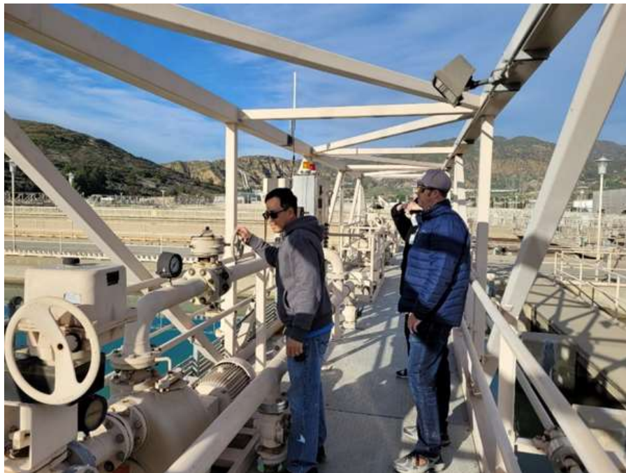
Staff removing settled solids from a basin using the traveling bridge control at the Jensen plant
