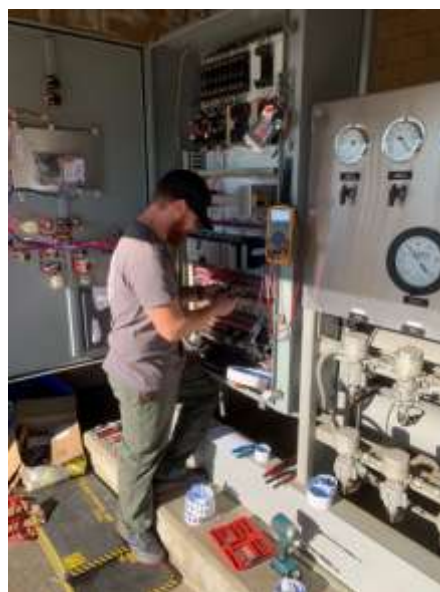
Staff installing programmable logic controller for the Secondary Inlet at DVL
