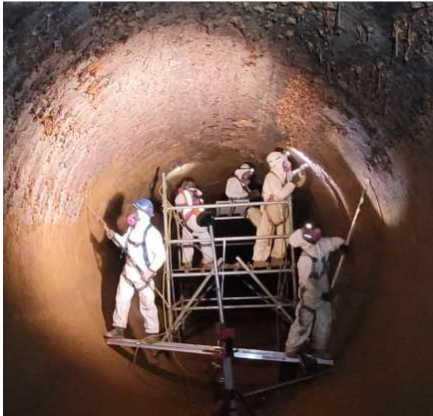
Etiwanda Pipeline Relining —Preparing pipe surface for relining
