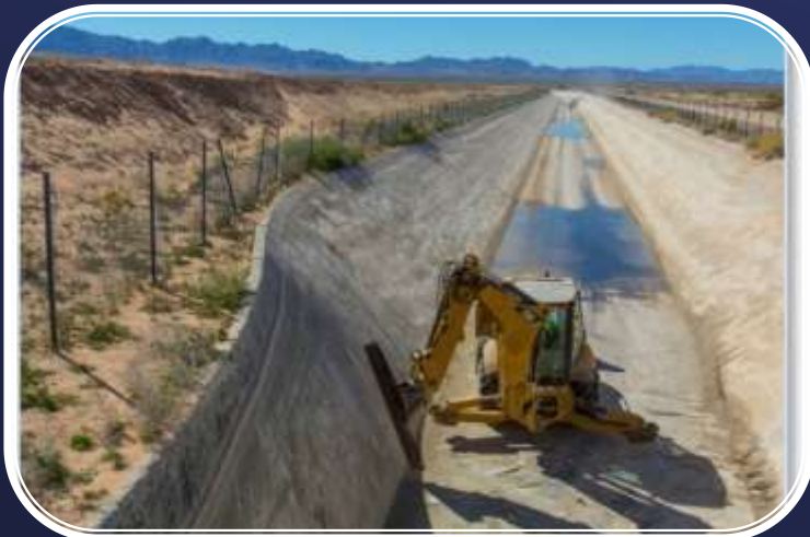
Desiccation, Cleaning and Inspections during CRA Shutdowns
