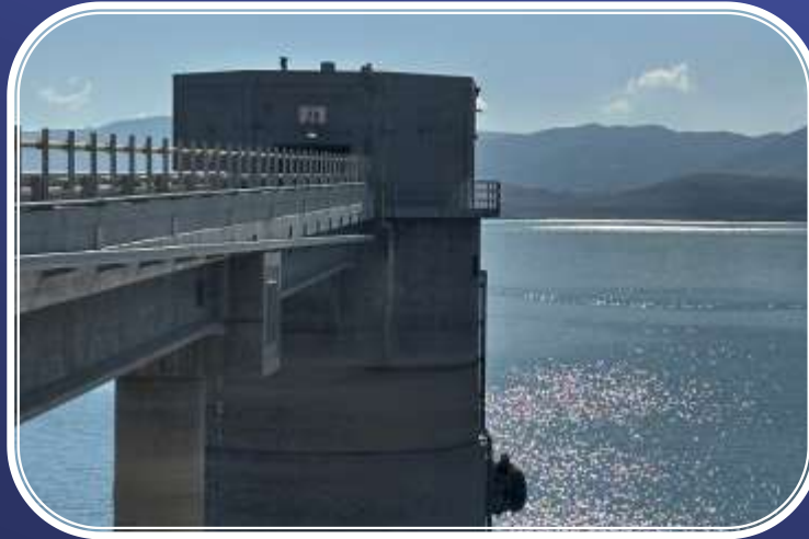
Periodic Tower Chlorination at Lake Mathews and Lake Skinner
