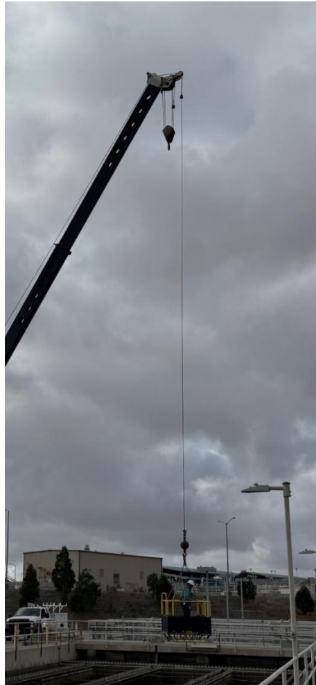
Staff working from utility basket to replace launders at Skinner washwater reclamation plant
