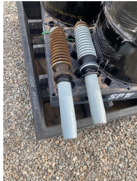
Gene-Peddler Line electrical testing and bushing replacement
