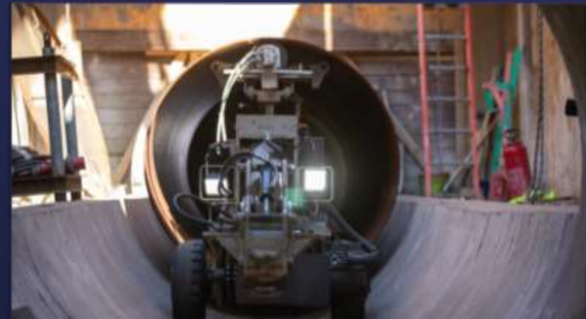
Second Lower Feeder
