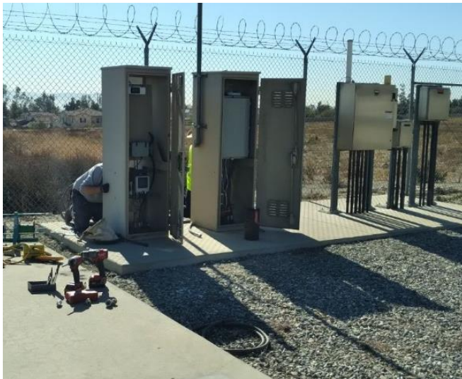
Staff modifying cabinets for the new communication equipment
