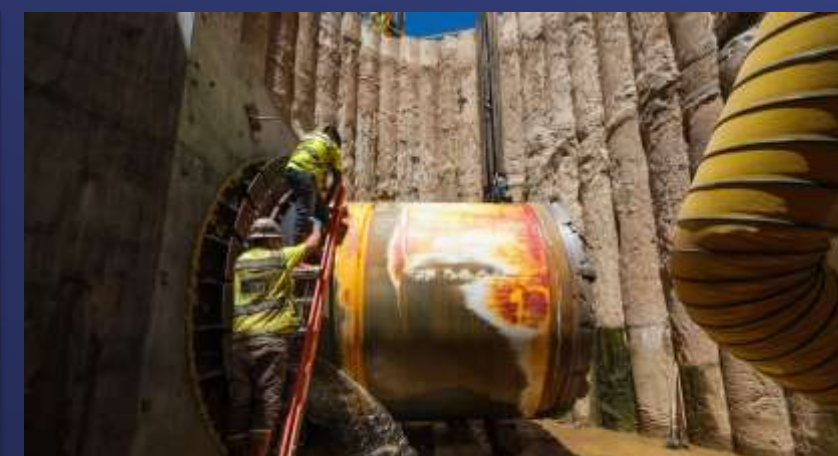
Perris Valley Pipeline
