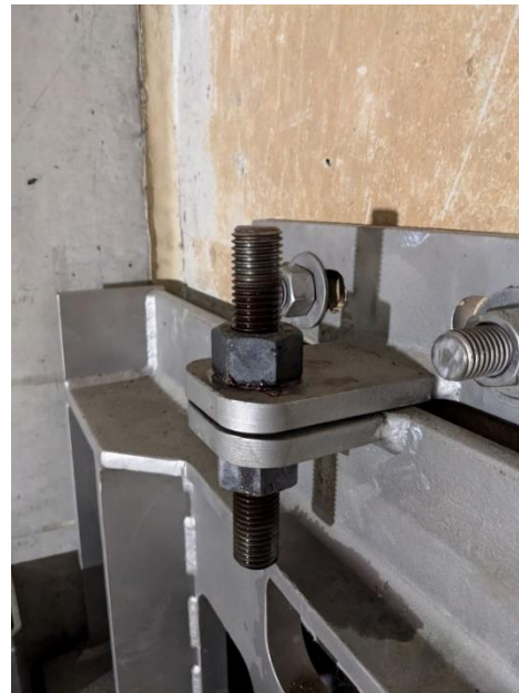
Weymouth rejection structure new door stop (left) and oversized hardware (right)
