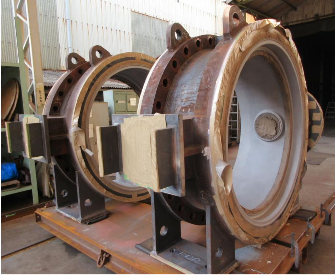
54-Inch Valve for Foothill Pump Station Intertie—Surface Preparation of Valve Interior before Rubber Lining
