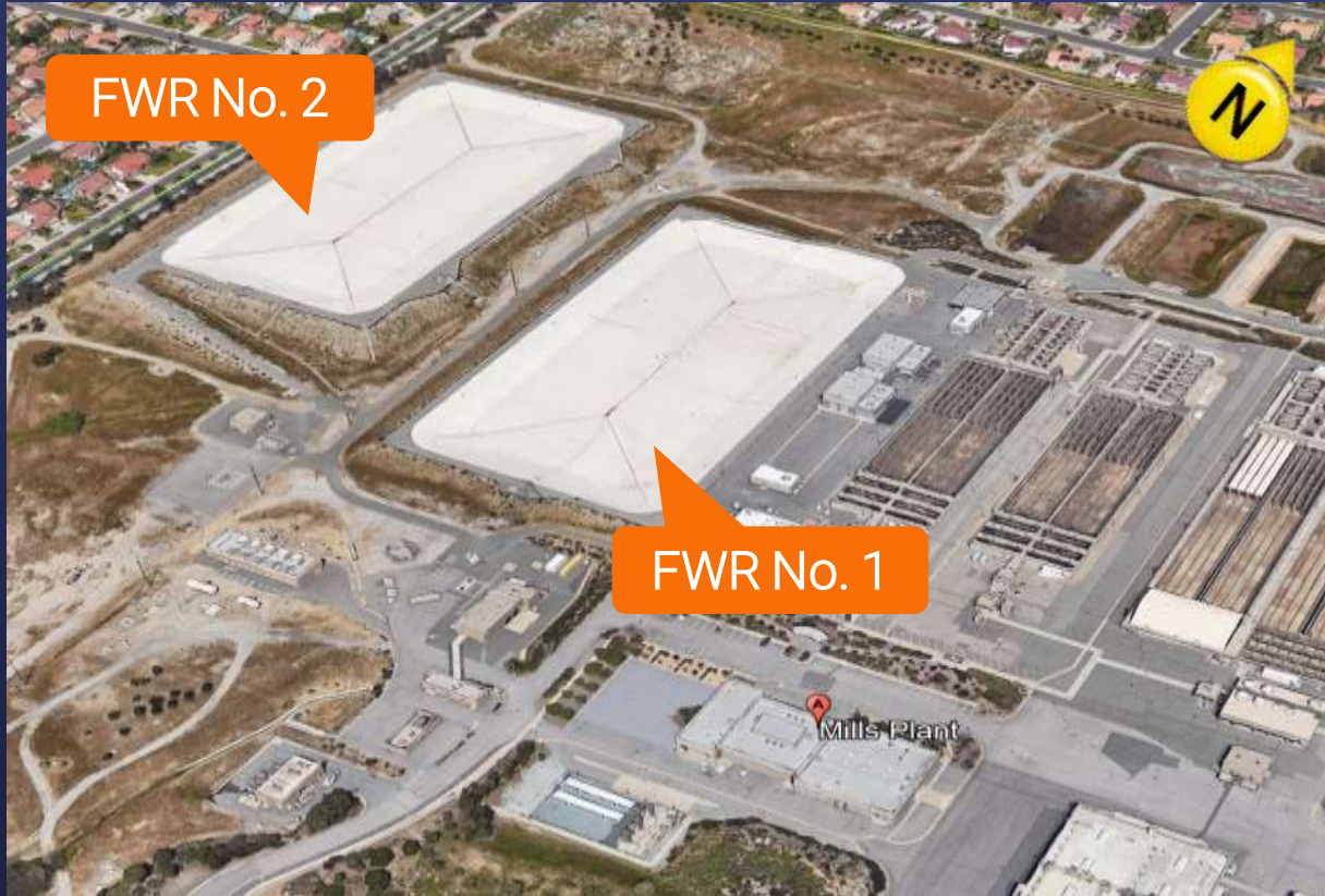
Henry J. Mills Water Treatment Plant
