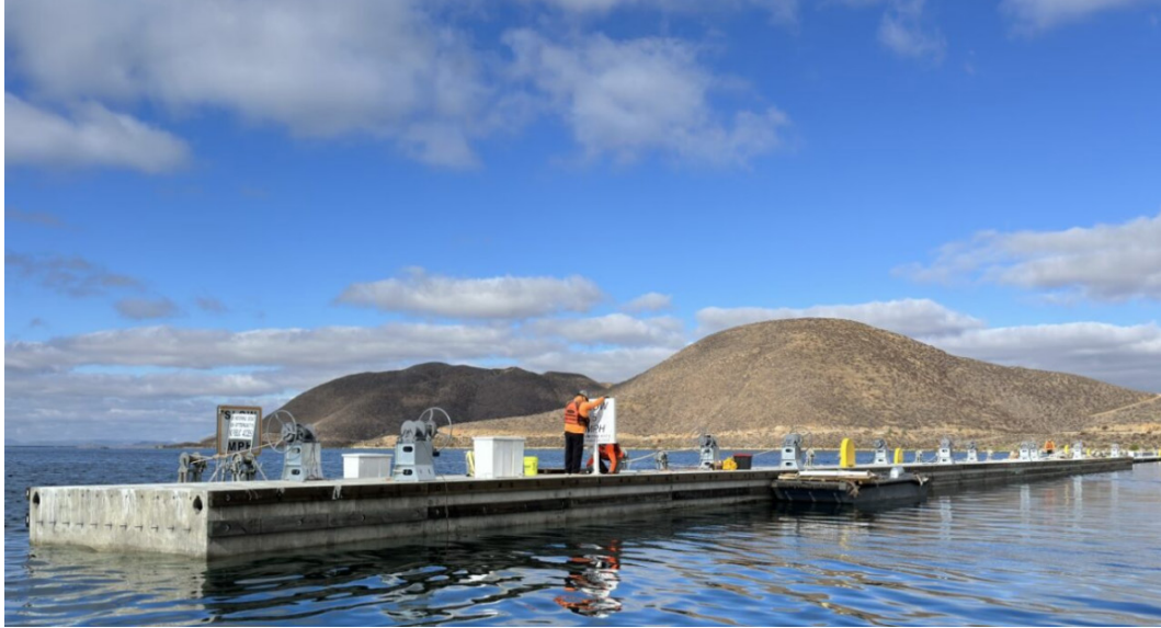
DVL FWA Replacement — Installation of Signage on North FWA
