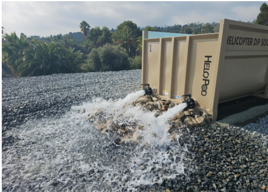
Palos Verdes Helopod Operational Testing
