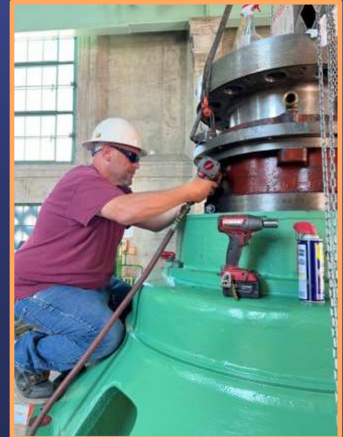
Iron Mountain – Working on the Pump Bearing Housing
