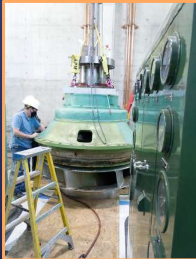
Iron Mountain – Impeller and Bearing Housing Removal
