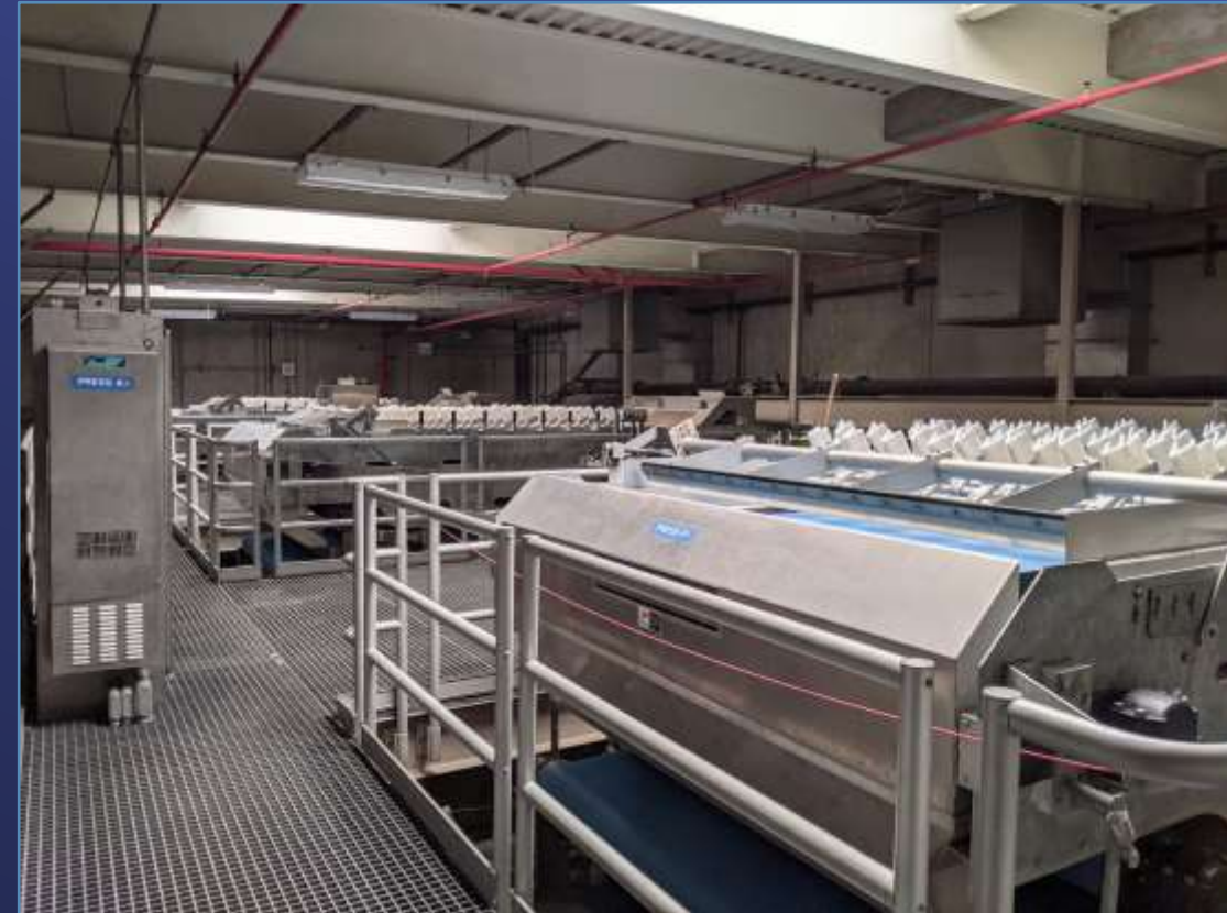
Mechanical Dewatering at Weymouth
