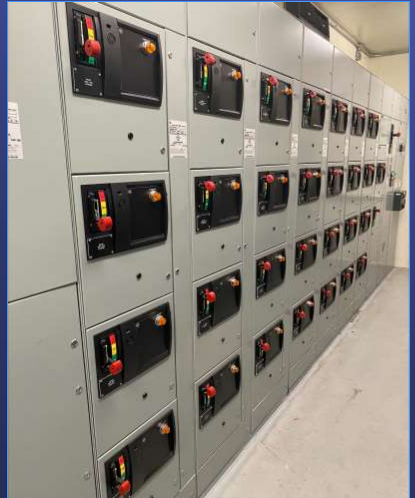
New UPC – Electrical Upgrades Stage 2
