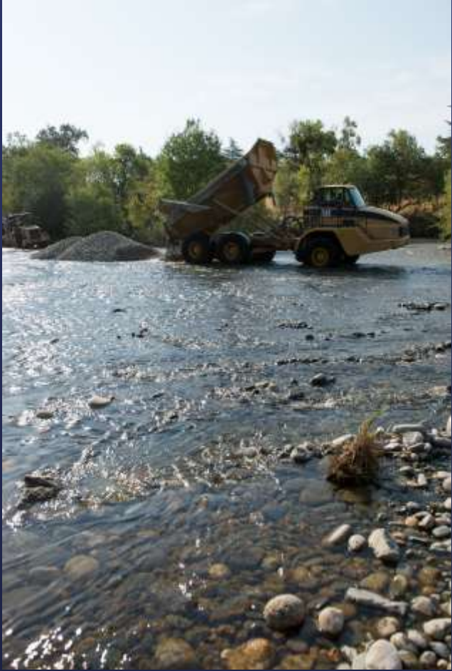
Spawning gravel augmentation on the Feather River. Photo Credit: The California Department of Water Resources
