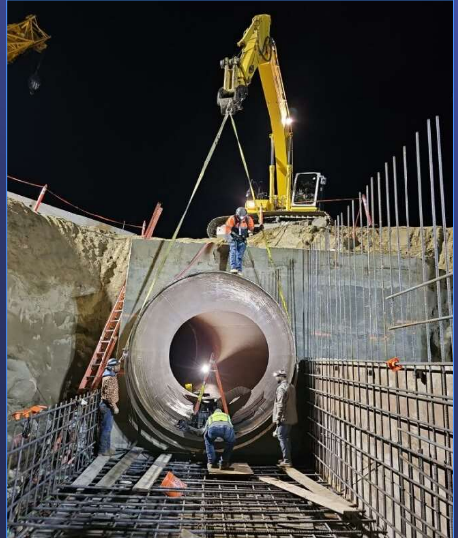
Wadsworth Bypass Shutdown work
