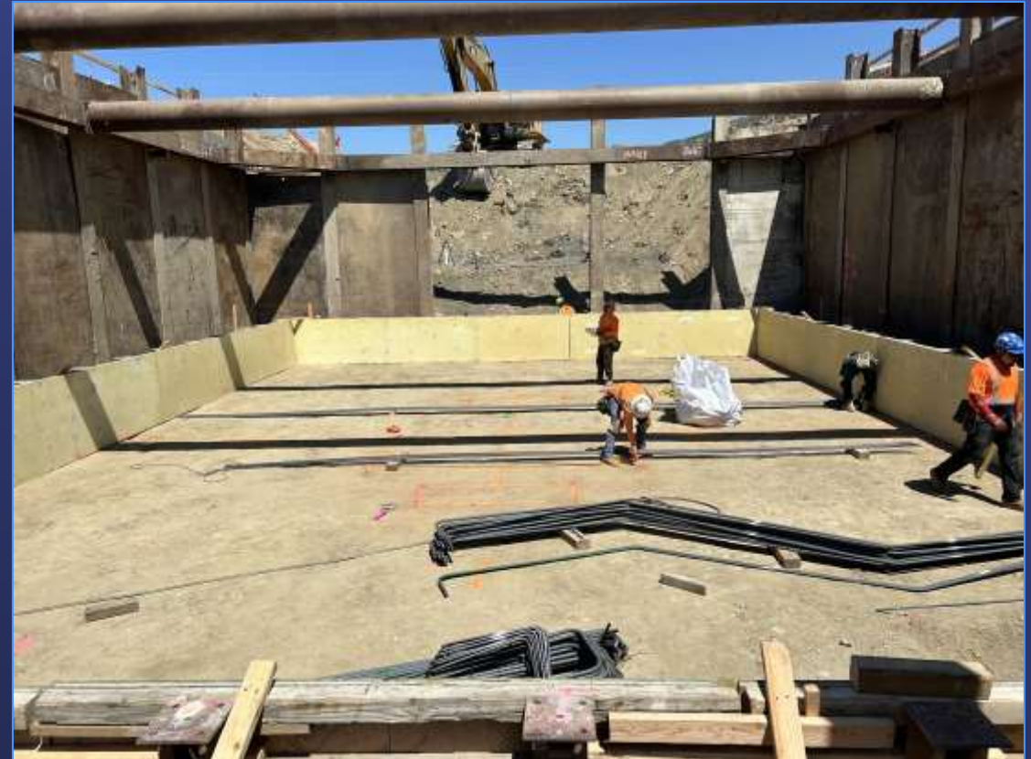
Preparation of Valve Vault Foundation
