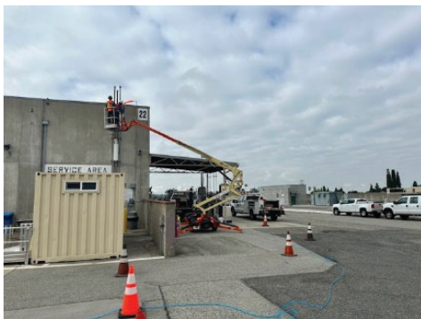
Vapor vent line removal above grade and capped
