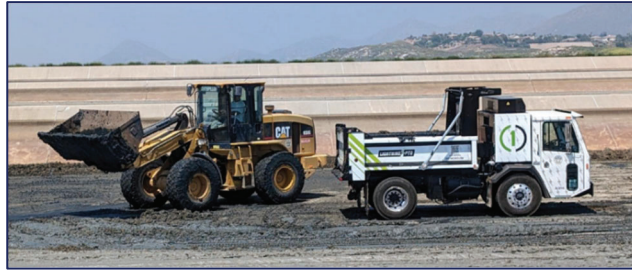
Battle Motors electric dump truck to transport sludge at Mills Plant
