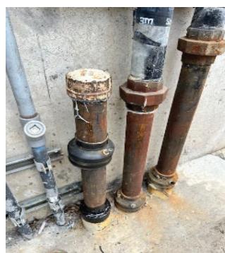
Vapor vent line removal above grade and capped
