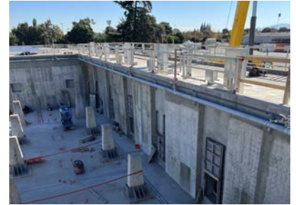
View of completed strengthening of basin walls
