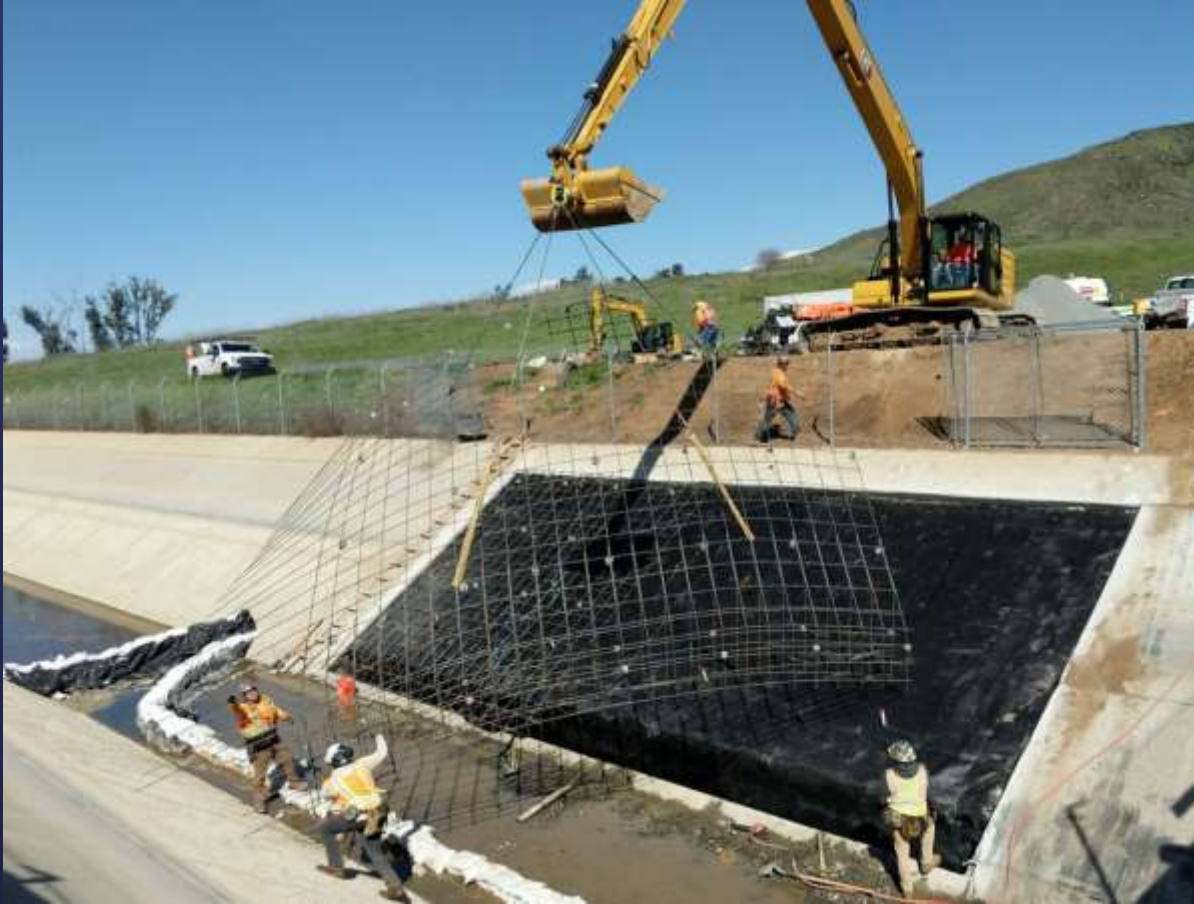
Reinforced Steel Installation
