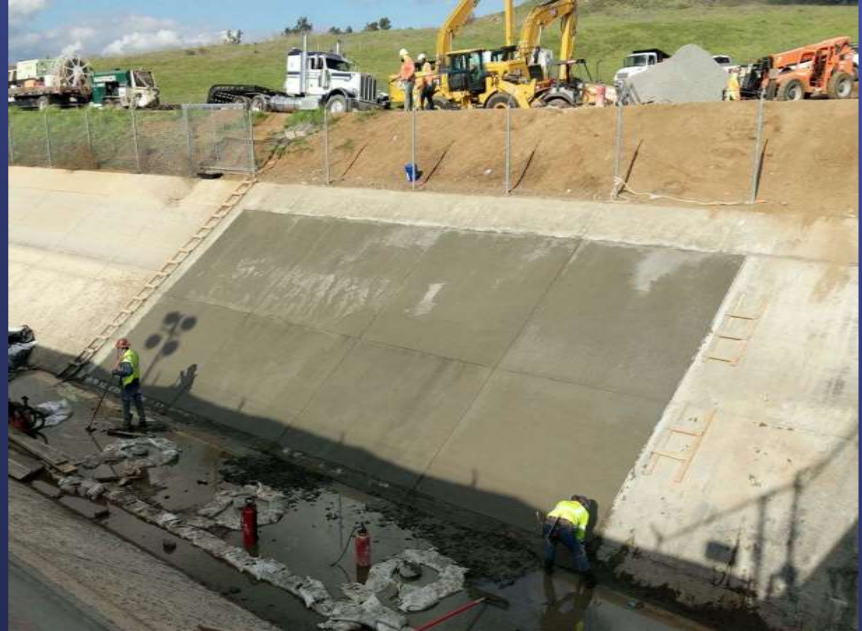
Concrete Panel Installation
