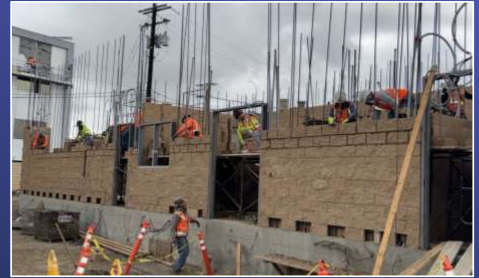
Venice PS Construction (June 2026)
