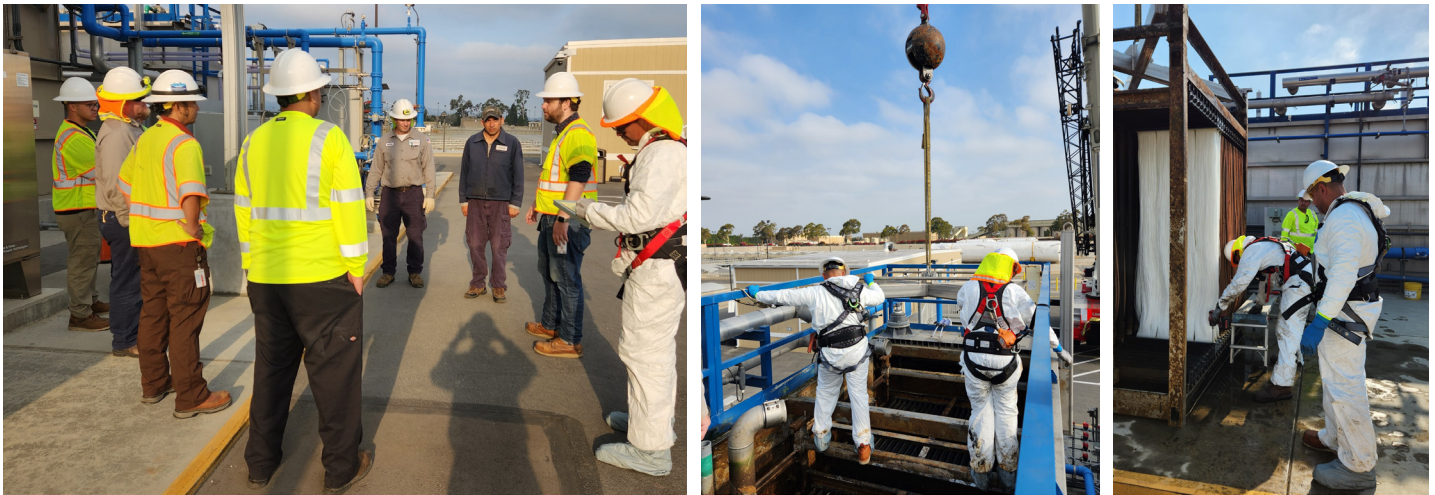
Metropolitan and LACSD staff in a safety meeting prior to MBR installation (left), using a crane to remove an MBR cassette (middle), and installing MBR modules (right)
