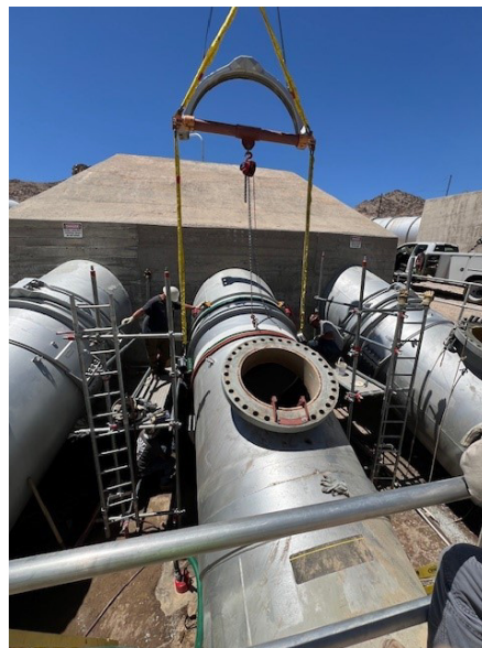
Staff remove pipeline isolator fitting from Iron Mountain Unit 5
