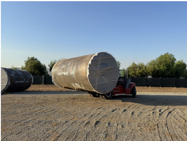
Staff unloading 120-inch diameter pipe (left) and pipe storage area (right)
