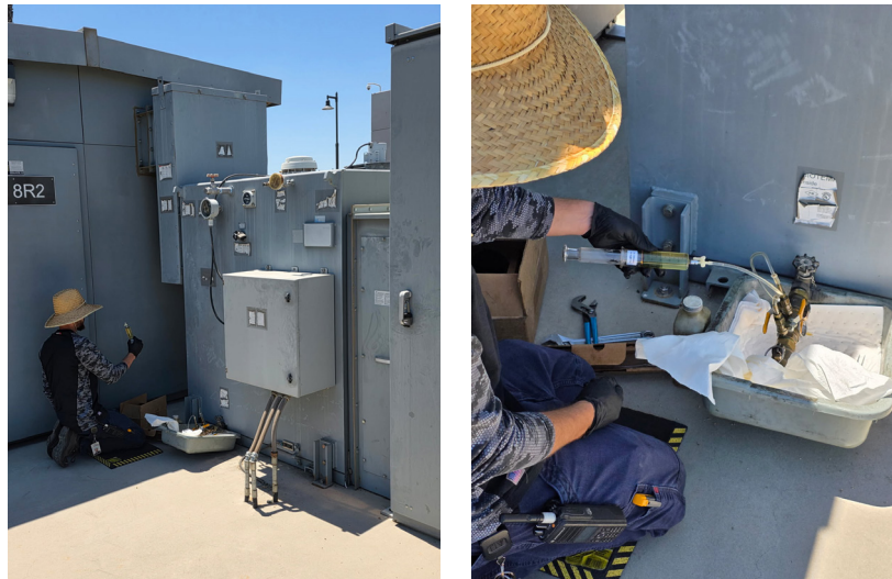
Oil-filled transformer (left) and taking an oil sample for dissolved gas analysis (right)
