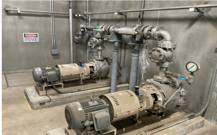
Repaired ozone analyzer sump pump system at Weymouth plant
