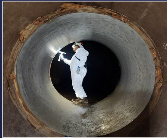
Mortar Lining Repair Inside the La Verne Tunnel
