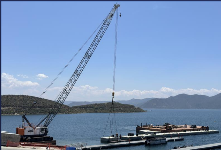
Hoisting Anchor Blocks into Water
