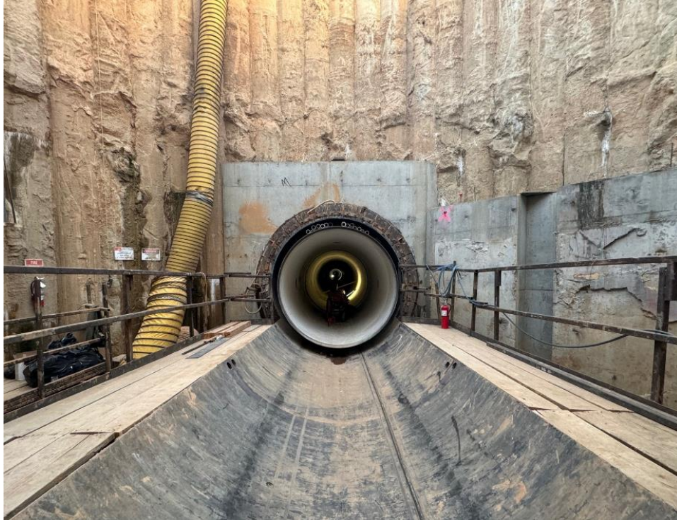
Perris Valley Pipeline Tunnels—Drive 2 Carrier Pipe Installation
