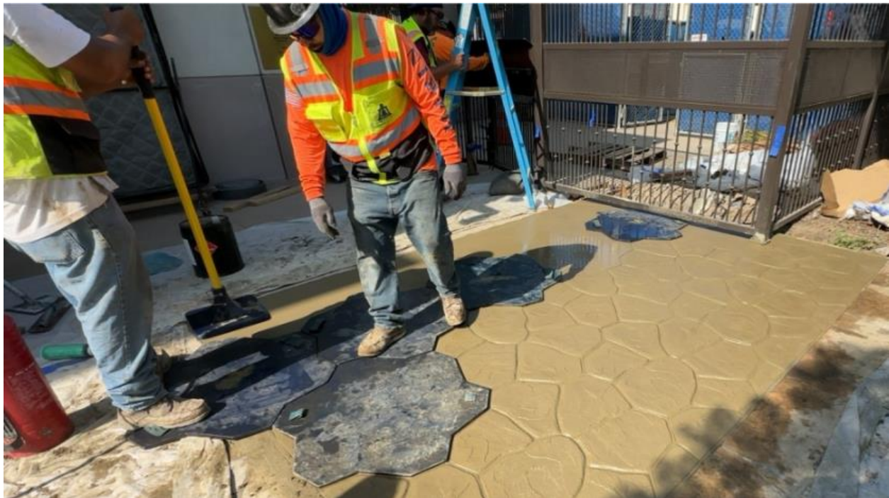
Headquarters Physical Security Upgrades—Stamping Concrete at Gate 4
