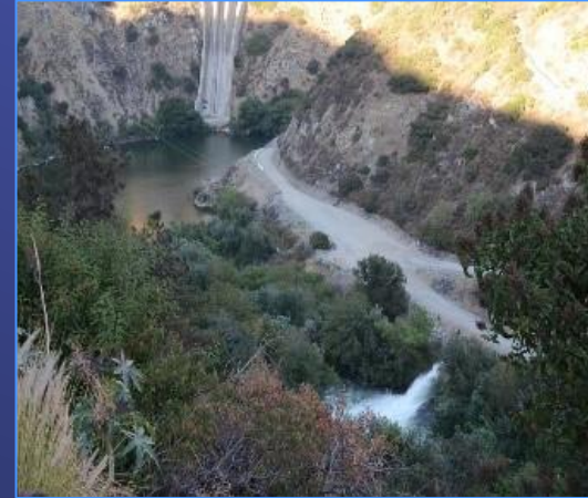
USG-03 Water Delivery
