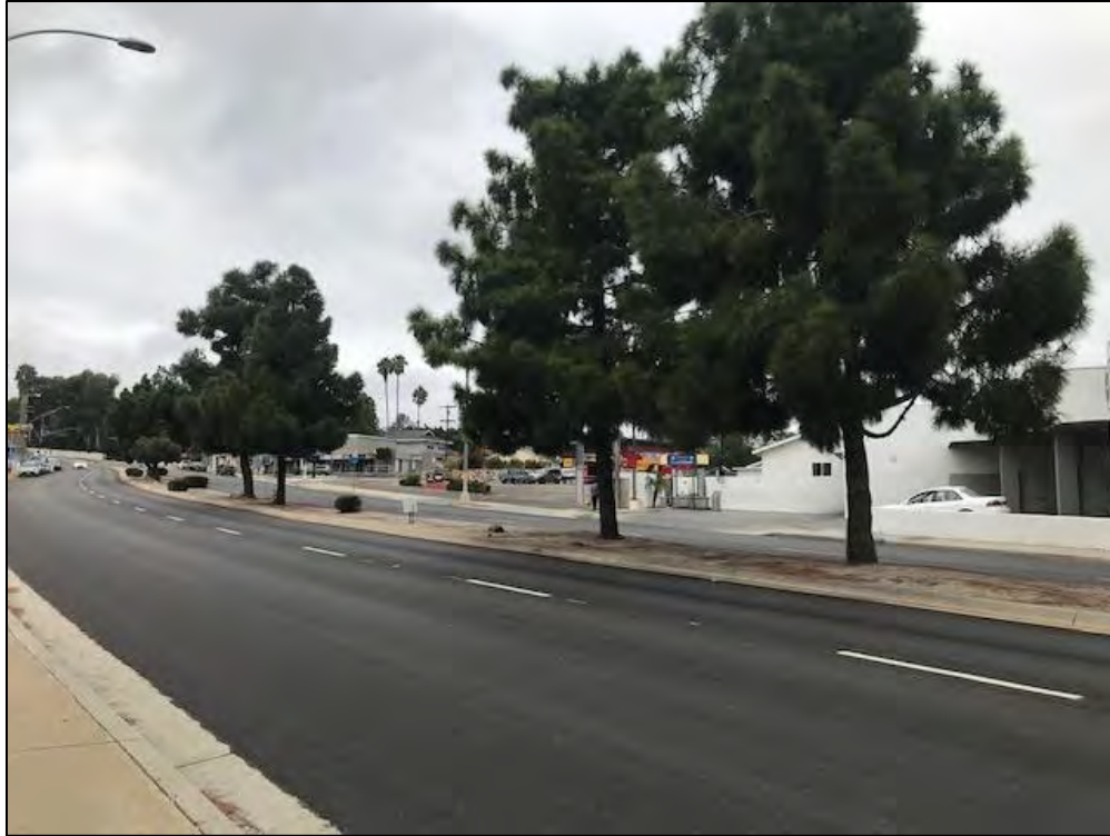
Photograph 5. Project site with street trees proposed for trimming/removal, facing south.
