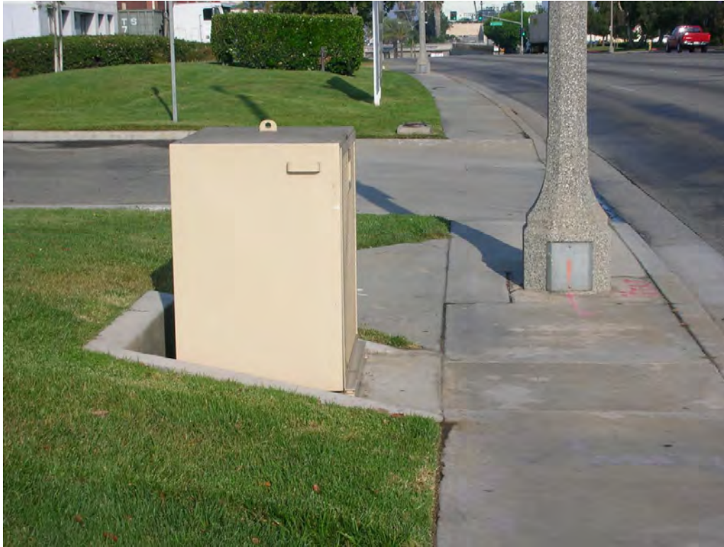
Figure 4. Typical Aboveground Valve Enclosure
