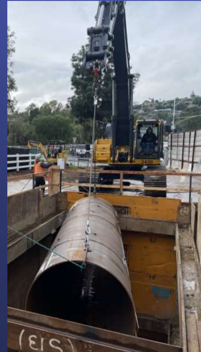
Second Lower Feeder Relining
