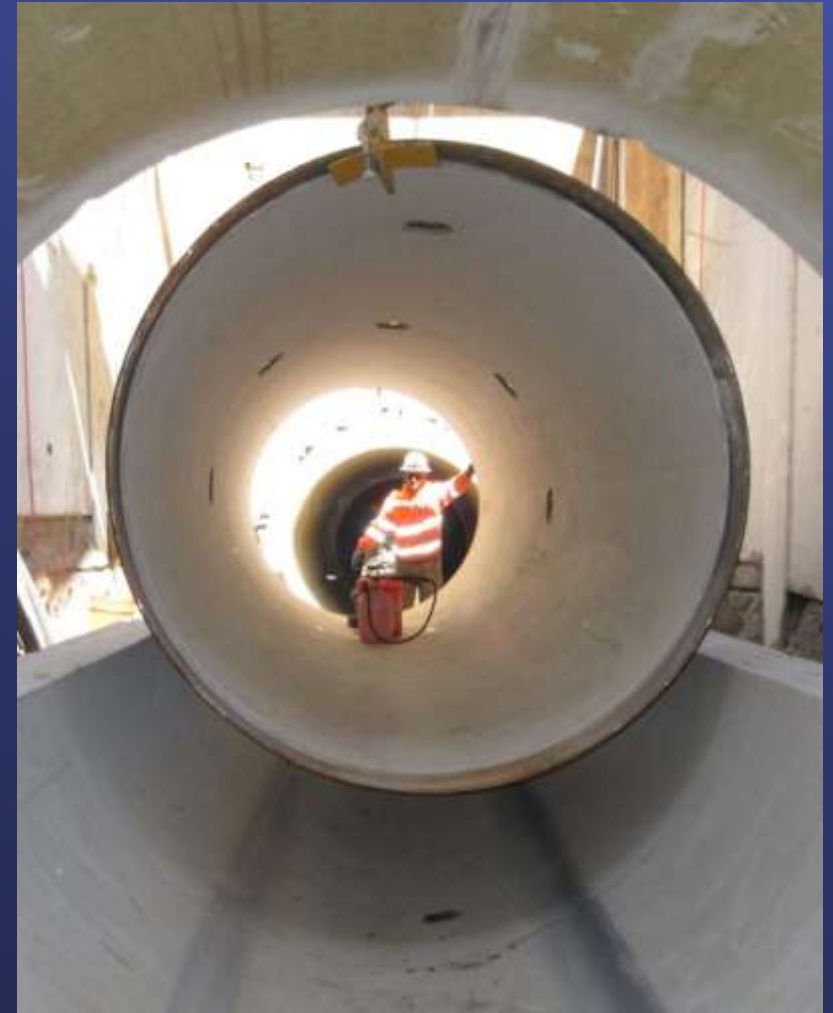
Allen-McColloch Pipeline Relining
