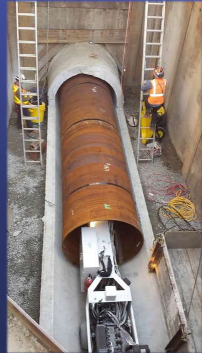
Second Lower Feeder Relining
