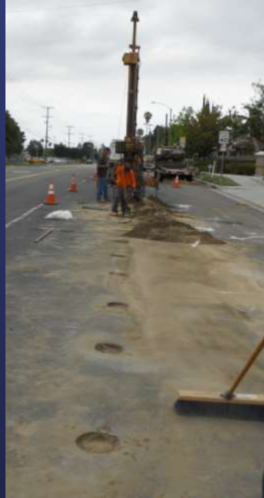
Drilling for Anodes
