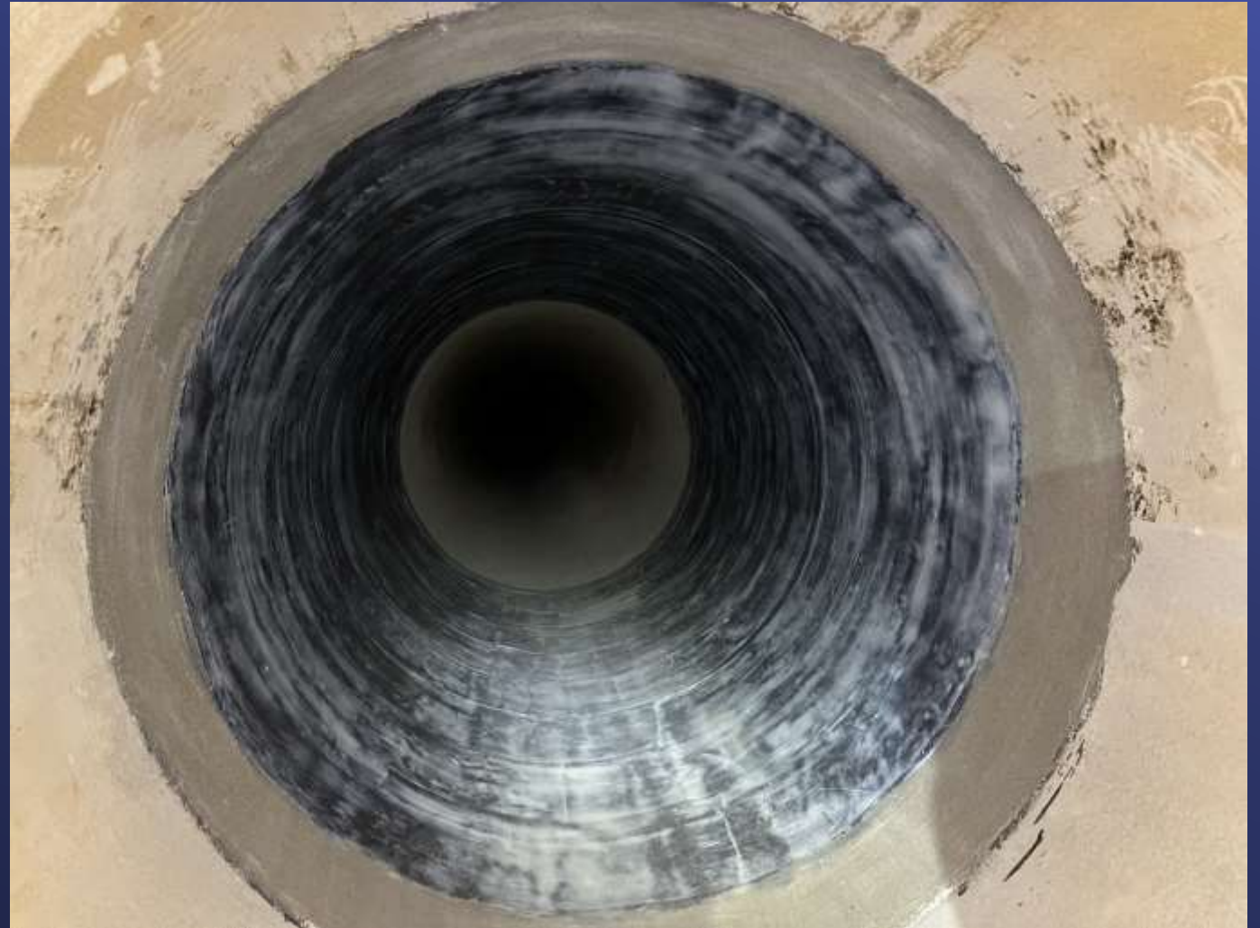
Sepulveda Feeder Urgent Carbon Fiber Lining
