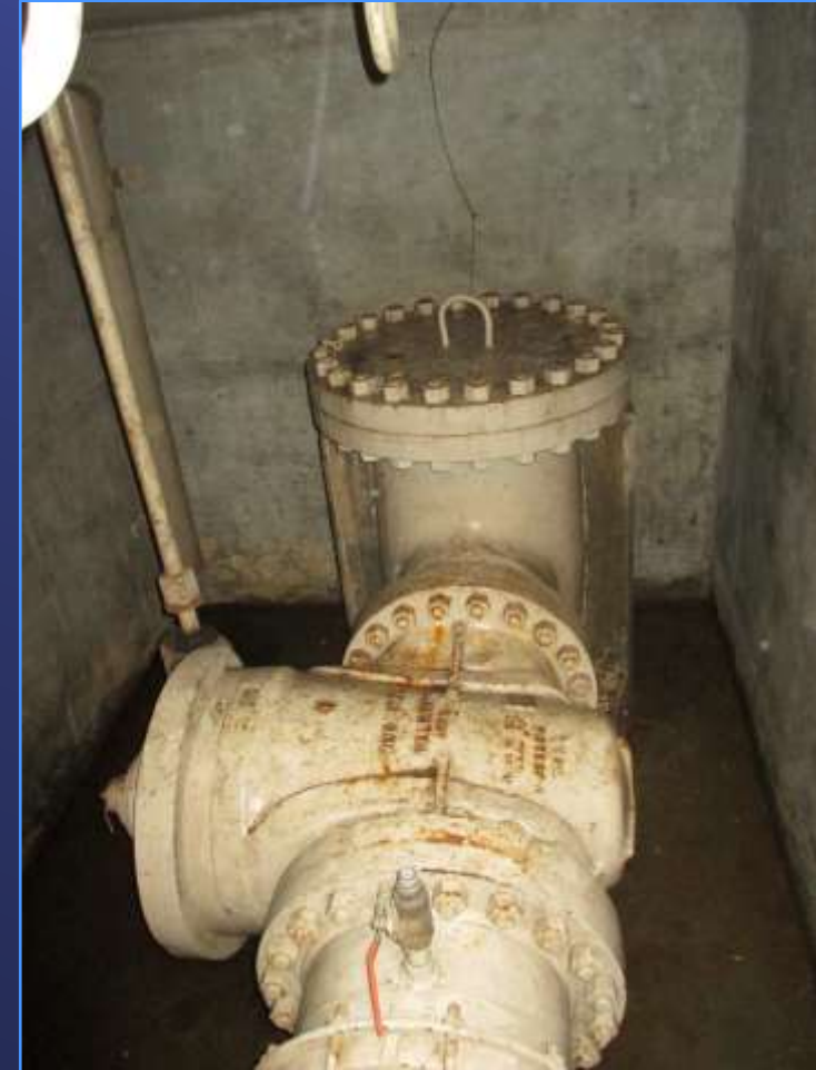
Existing deteriorated blow-off valve, typical of six
