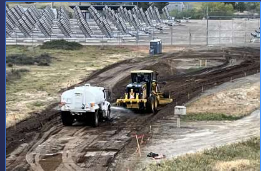
Skinner Plant Battery Project Site Prep
