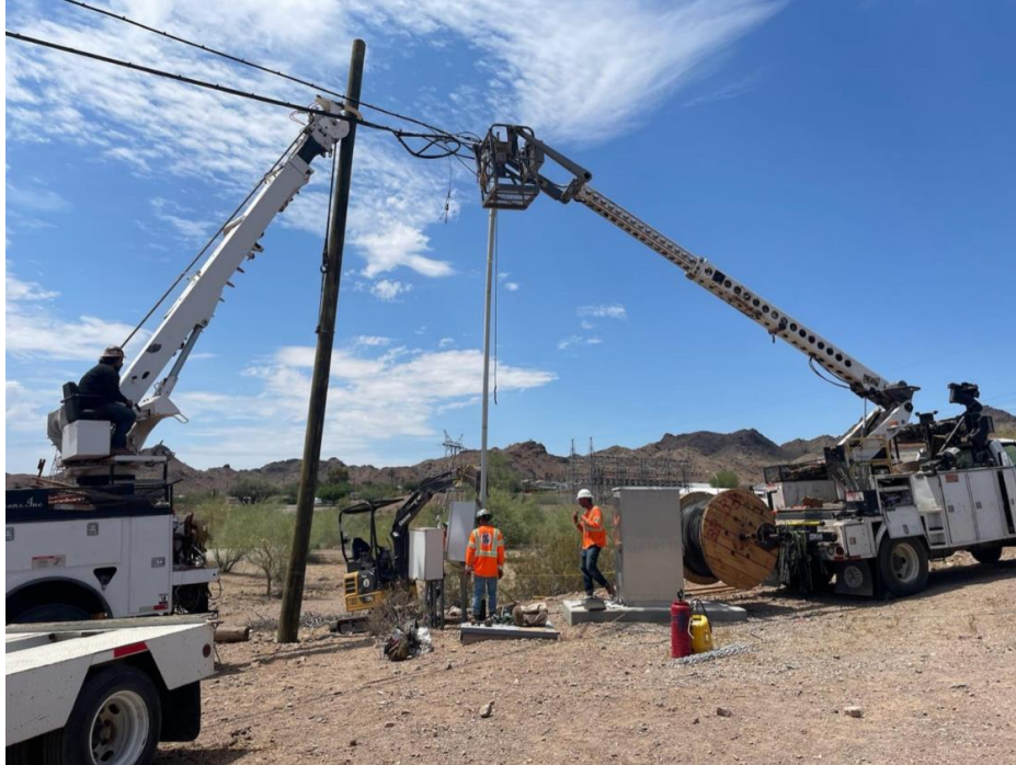
Gene Communications System Upgrade – Pole #1 Replacement
