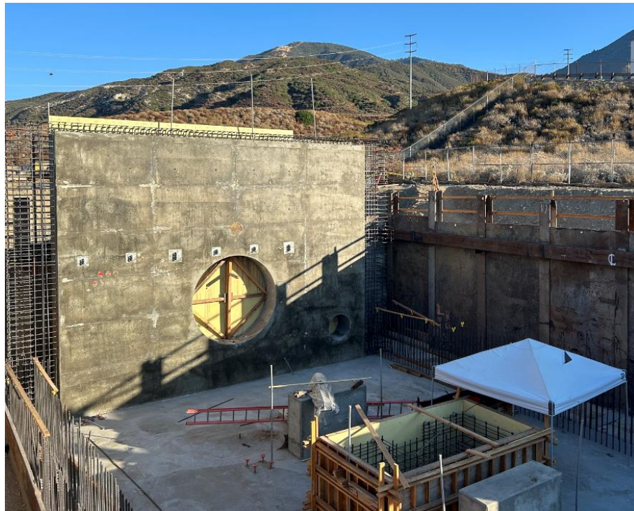
Inland Feeder-Rialto Pipeline Intertie – Valve Vault Wall Complete – Looking West
