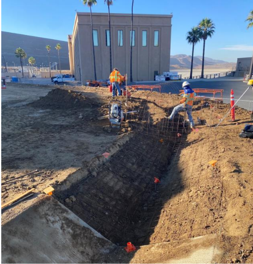
Wadsworth Pumping Plant Bypass – Placing Rebar Wire Mesh for V-ditch
