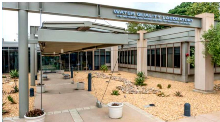
Main Entrance to Water Quality Laboratory Building
