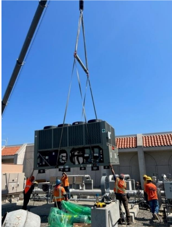
Service Connection OC -88 Chillers Replacement – Chiller Installation
