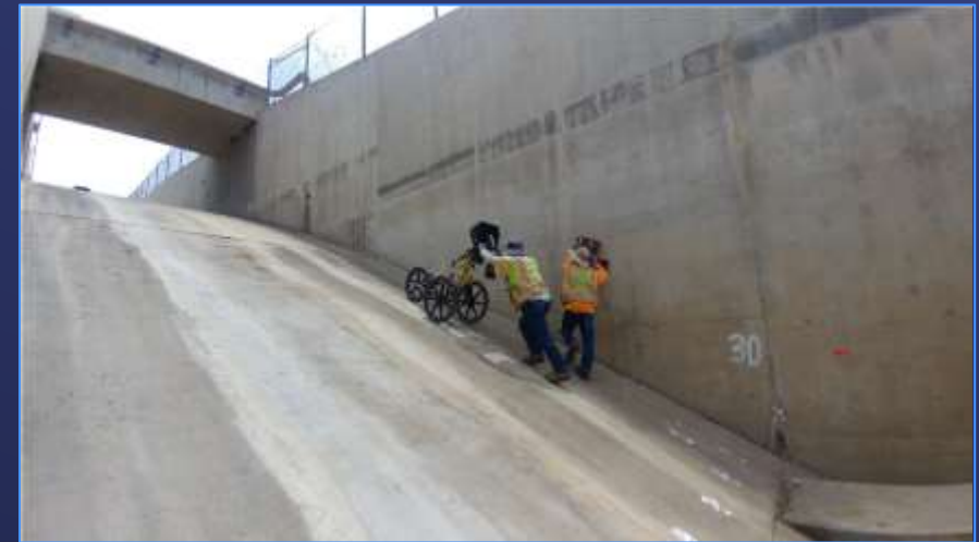
Lake Skinner Spillway GPR Testing
