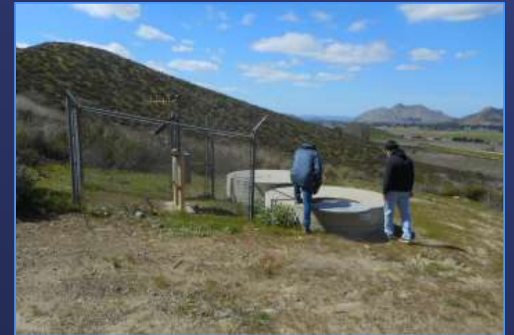
DVL Seepage Monitoring Station
