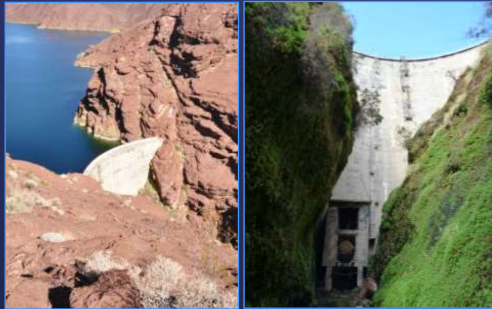
Copper Basin Dam
