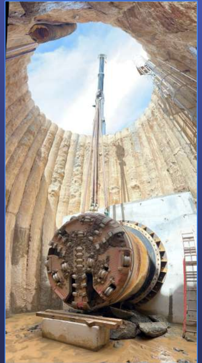
Perris Valley Pipeline Construction
