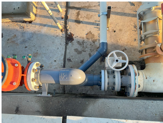
Newly installed reducing flange, valve, and PVC piping
