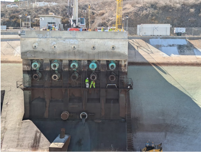
Staff working at the forebay (left) and inspecting the large 10-foot wide isolation gate at the junction shaft at Lake Mathews (right)
