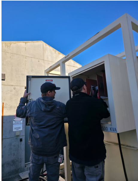
Staff making transformer connections (left) and generators and transformer being staged for service (right) for testing of an Emergency Power System at Weymouth plant
