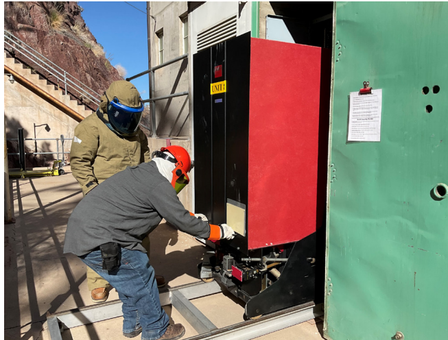
Staff prepares a 6.9kV circuit breaker for maintenance at Intake pump plant
