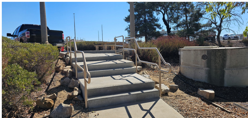
Newly upgraded stairs at the Skinner plant parking lot
