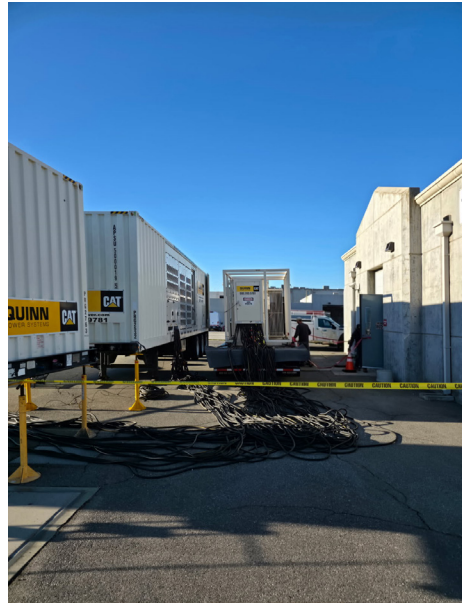
Staff making transformer connections (left) and generators and transformer being staged for service (right) for testing of an Emergency Power System at Weymouth plant
