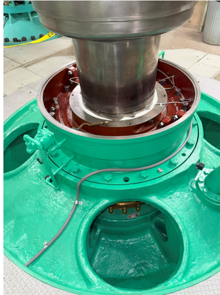
Eagle Mountain pump plant Unit 9 rehabilitation
