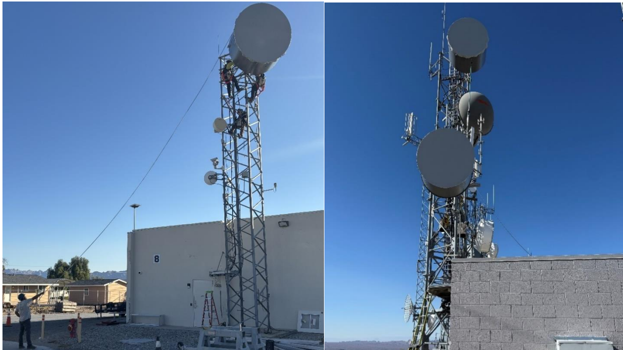
Installation of microwave antenna and waveguide on existing communication tower at Eagle Mountain Pumping Plant (left) and Chuckwalla site (right)
