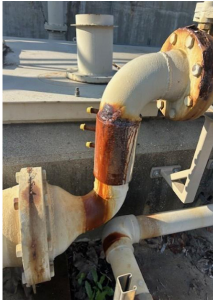
Corroded and patched piping (left) and newly fabricated and coated reducing flange (right) for the Weymouth industrial water system
