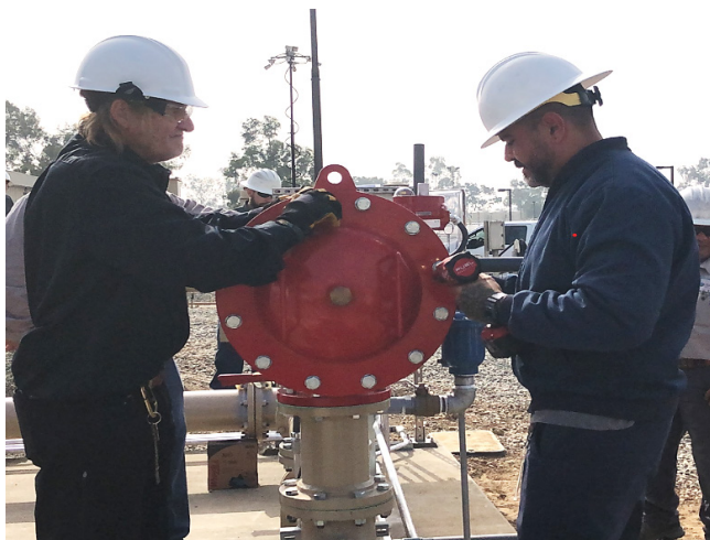
Staff working with vendor and LACSD research partner to install snail mitigation equipment at the demonstration facility
