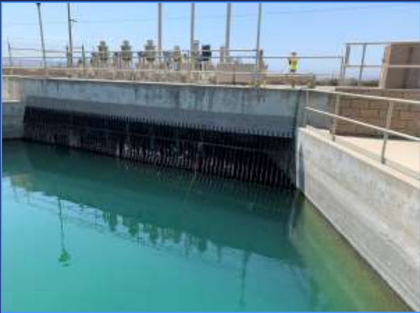
Bypass Channel Inlet
