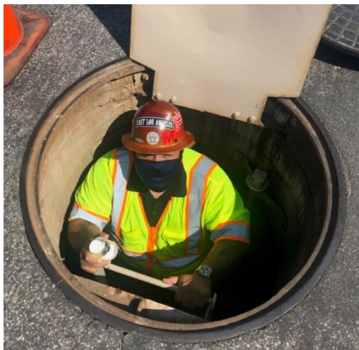
Engineer Victor Galvez working a pipeline shutdown
