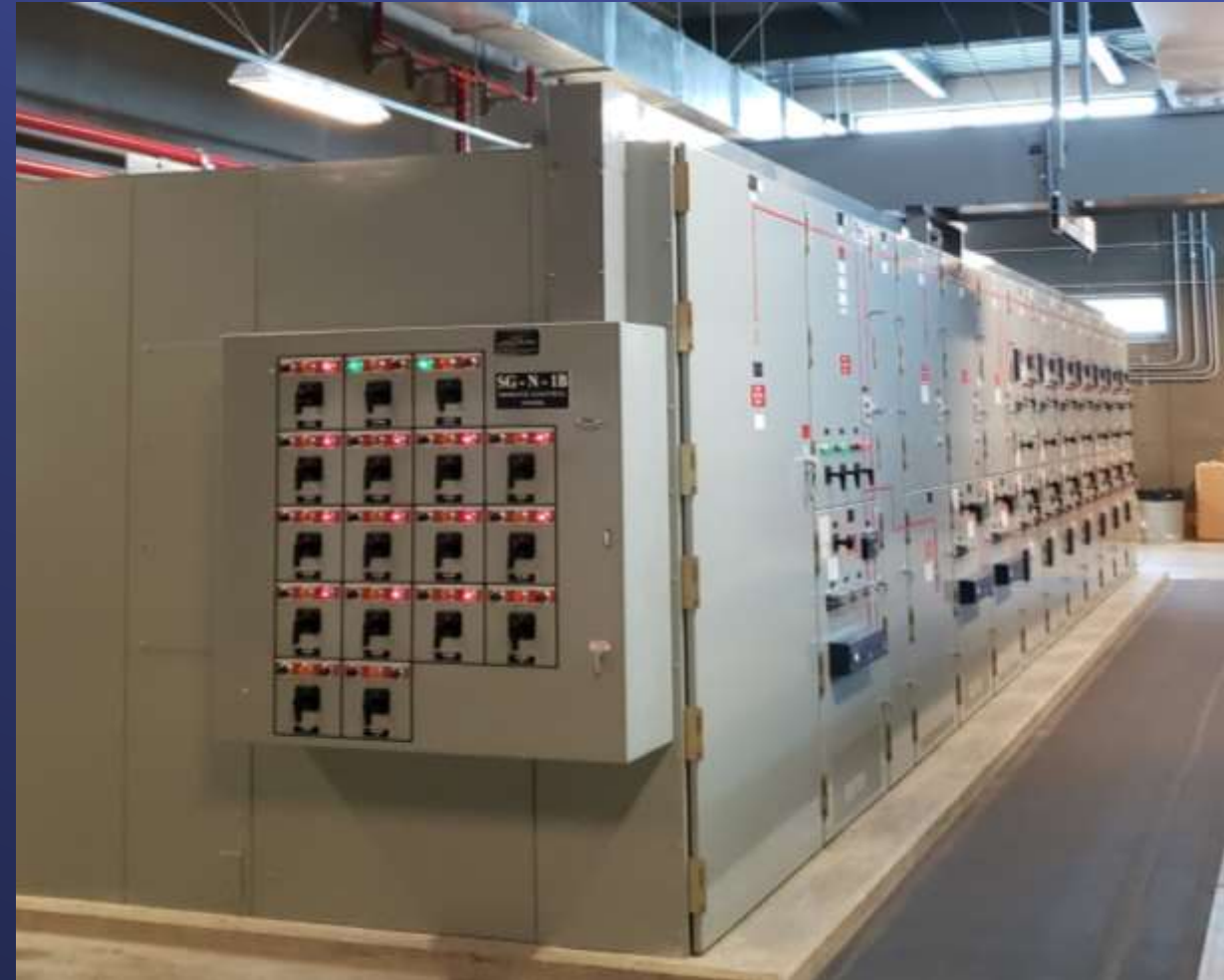
Proposed Indoor 4.16 kV Switchgear
