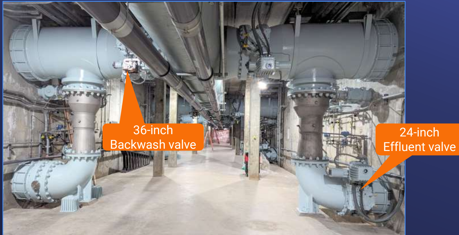
Weymouth Filter Building No. 2
