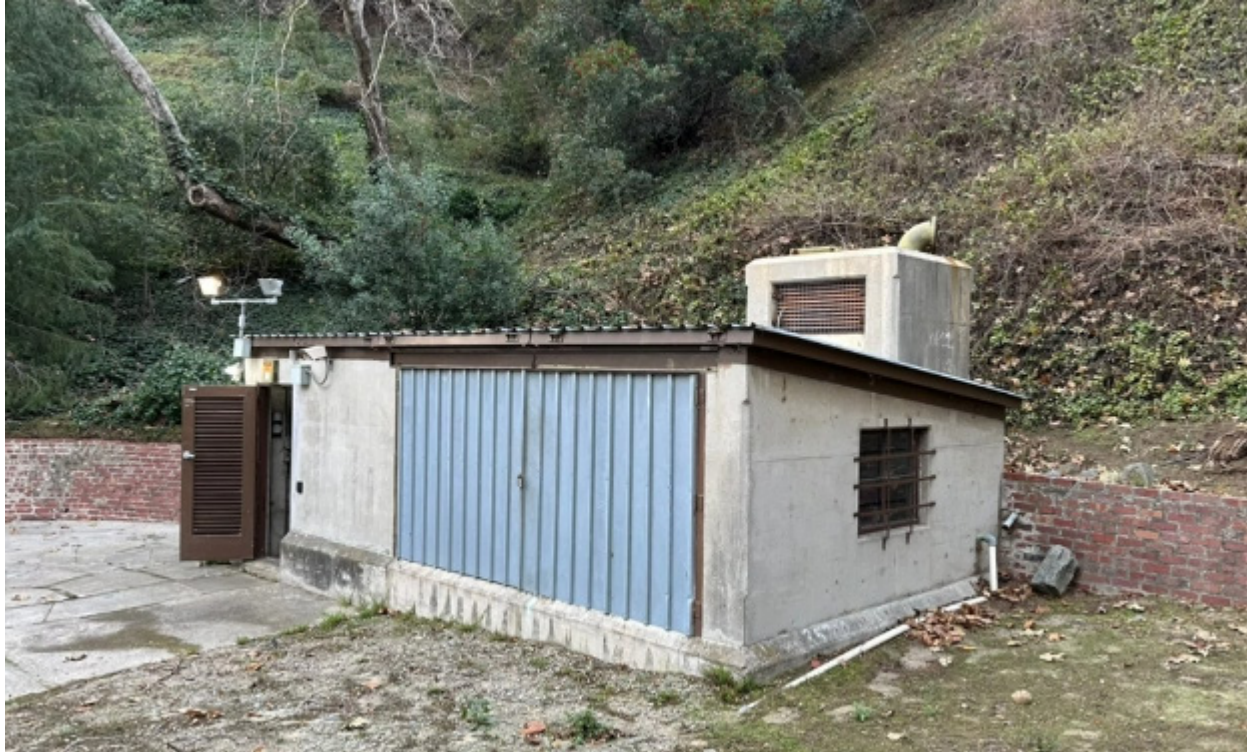
Hollywood Tunnel North Portal Control Structure
