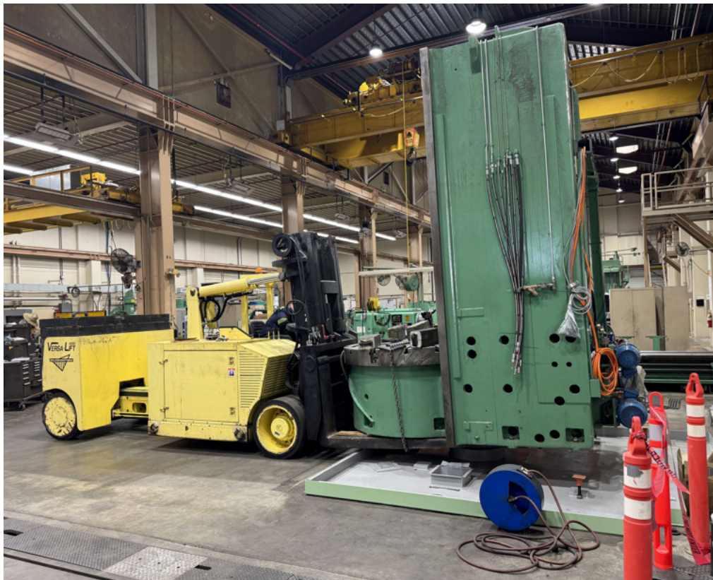
La Verne Shops Improvements — Installing Refurbished Vertical Turning Lathe Main Assembly at Fabrication Shops
