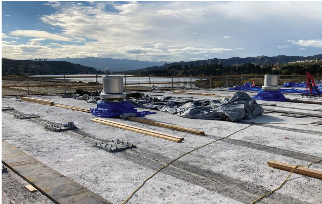
Installation of steel reinforcement plates on roof of the Foothill Hydroelectric Power Plant building
