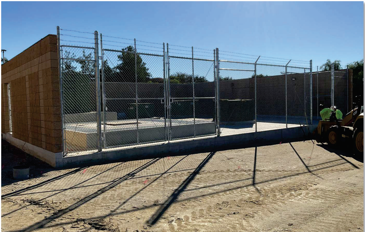
Expanded Riverside Public Utility switchyard for the second utility service for the Mills plant
