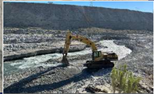
Whitewater River Repairs
