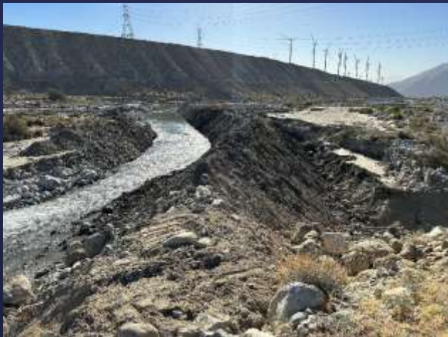
Whitewater Channel Repair
