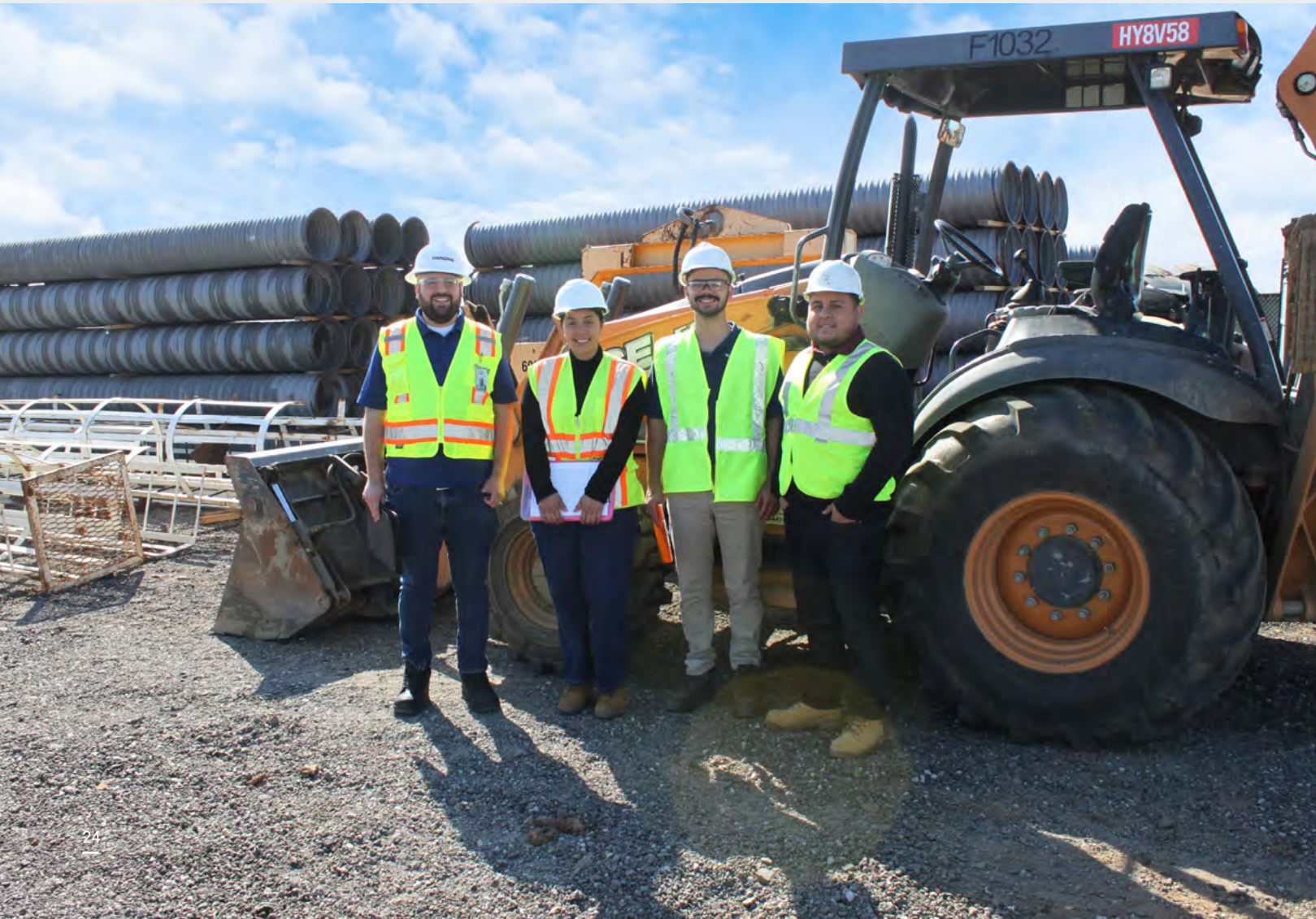
Project Labor Coordinator team meets with labor compliance consultant Alliant Consulting at the Perris Valley Pipeline Interstate 215 Crossing project. Pictured left to right Thomas Romero (Parsons Corporation), Kiara Salto, Troy Baggott and Diego Anaya (Alliant Consulting).
