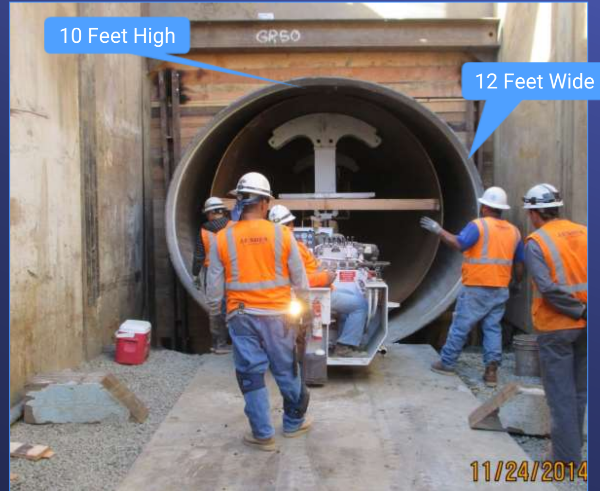
Bernasconi Tunnel Lining
