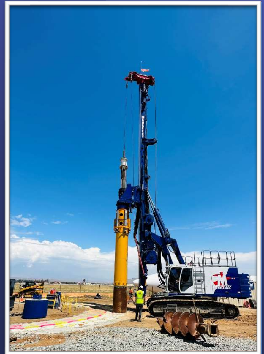
Perris Valley Pipeline I-215 Project
