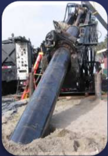
Slant Well Construction
