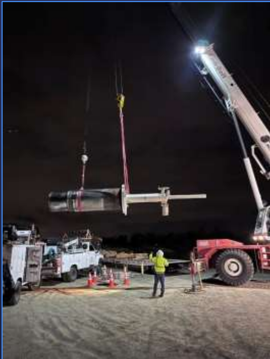
Sleeve valve assembly w/ actuator
