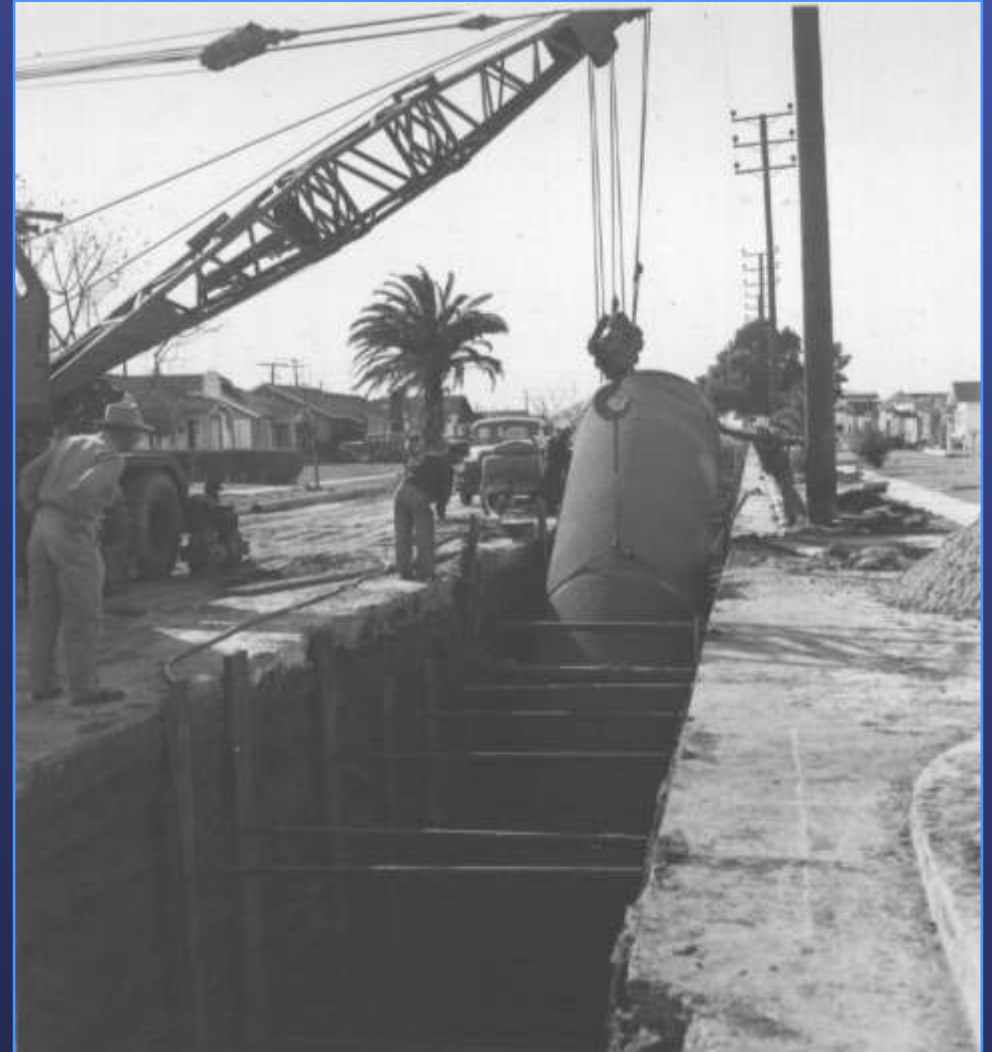
Middle Cross Feeder Construction - 1955
