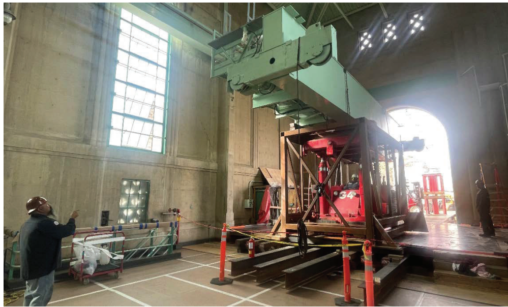
Installing the overhead crane girder at Eagle Mountain Pumping Plant
