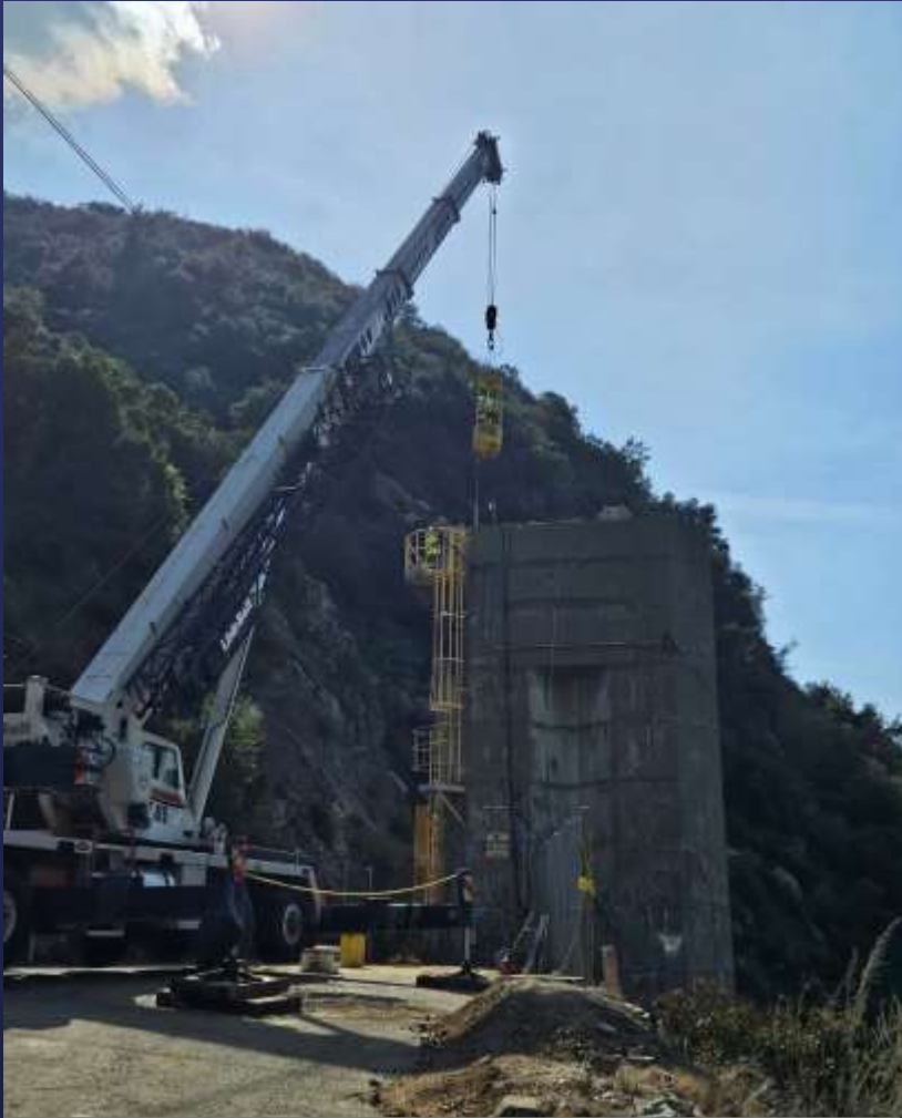
Crane Support – San Gabriel Tower
