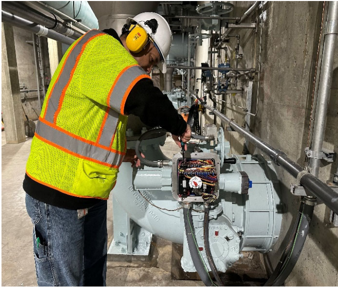
Staff adjusting valve position indicators (left) and verifying panel indication (right) at Weymouth plant
