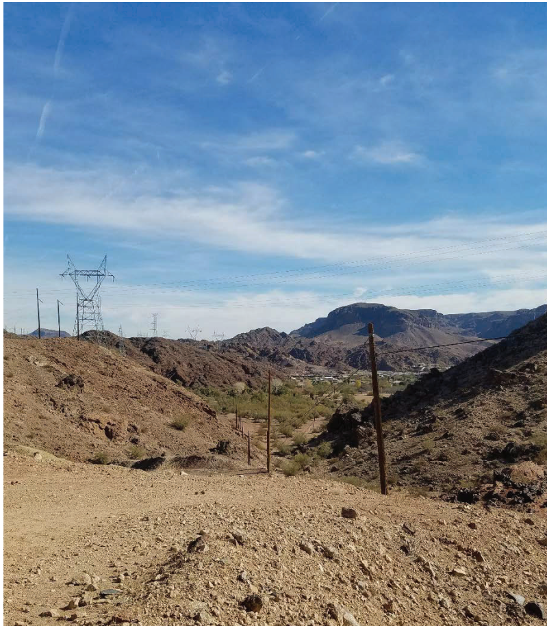
Existing communication line on wooden poles
