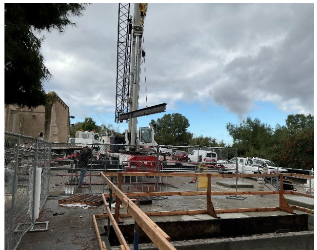
Staff mounting I-Beams to structure walls (left) and 100-ton crane hoisting I-Beams (right) at OC-88 valve structure along the AMP
