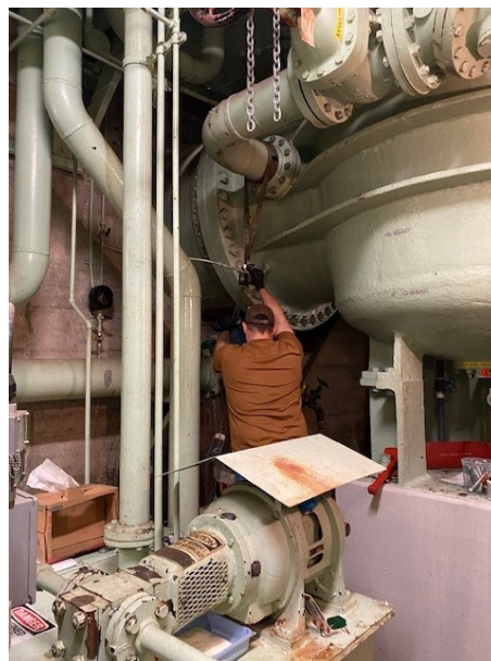
Staff replacing a circulating water supply valve at Gene pumping plant
