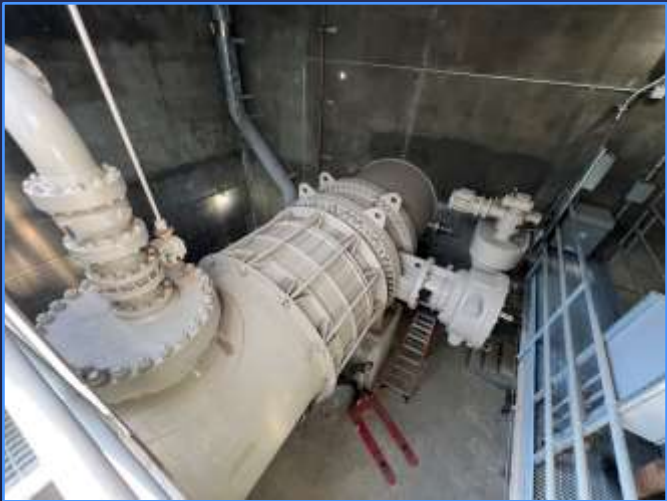
Typical Butterfly Valve & Actuator
