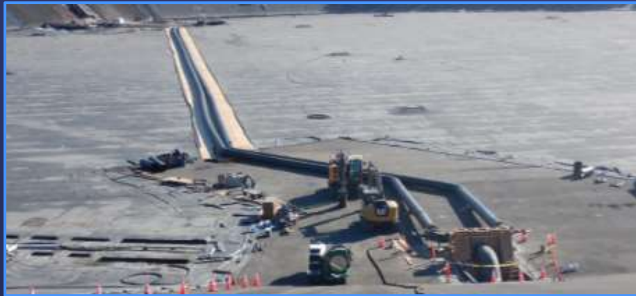
Completed 28-inch HDPE bypass at Palos Verdes Reservoir
