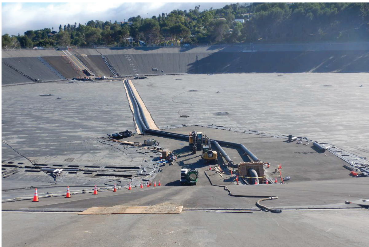
Completed 28-inch HDPE bypass at Palos Verdes Reservoir
