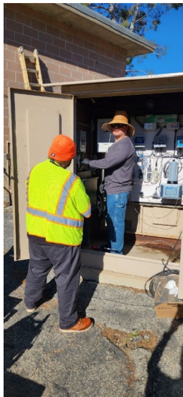
Staff installing a new water quality panel at Palos Verdes Reservoir
