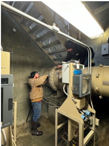
Staff performing venturi meter maintenance at the Skinner plant
