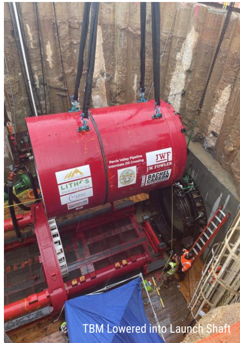
Tunnel Launch Shaft
