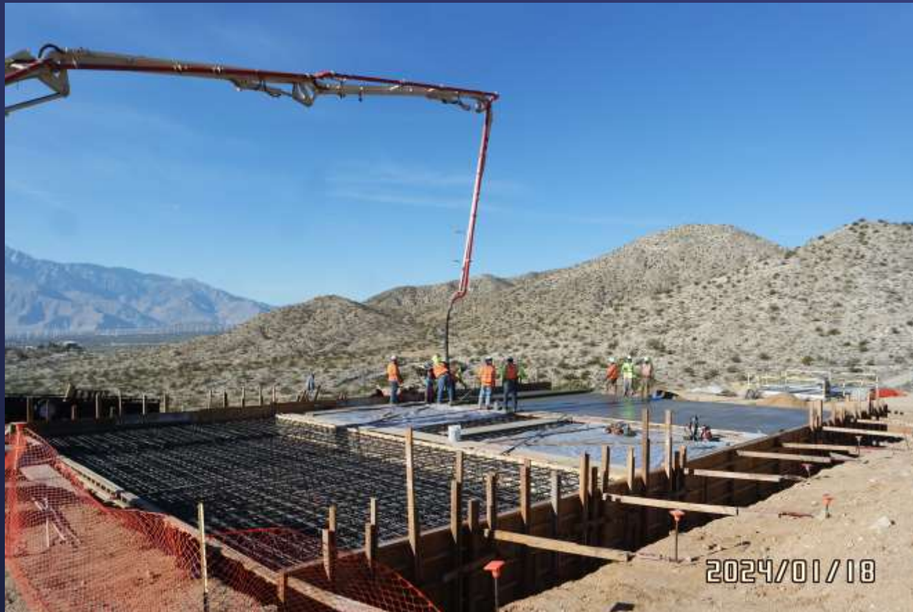
Placement of concrete for protective slab above aqueduct
