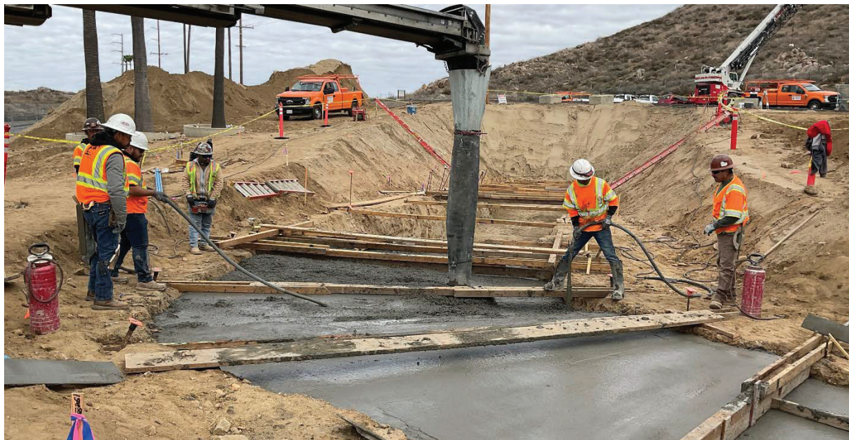
Placing concrete pipeline encasement for 96-inch diameter bypass pipeline
