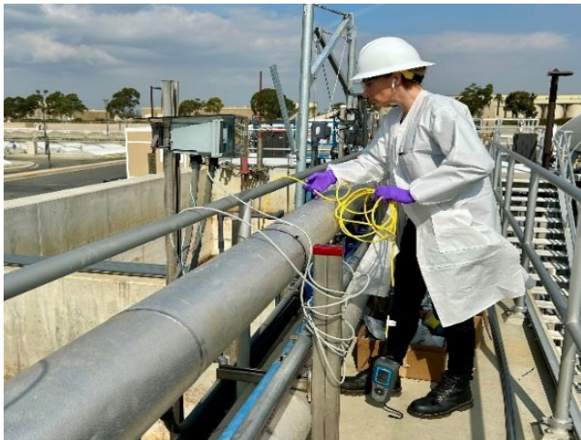
Dissolved oxygen measurement in the NIC demonstration facility bioreactors
