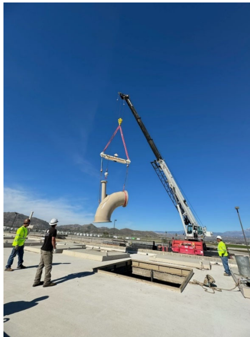
Staff reinstalling a sleeve valve at PC-1 Pressure Control Facility
