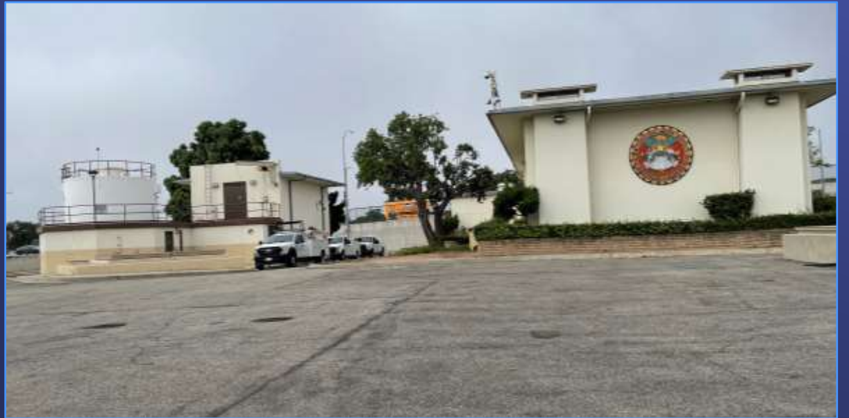
Venice Hydroelectric Plant
