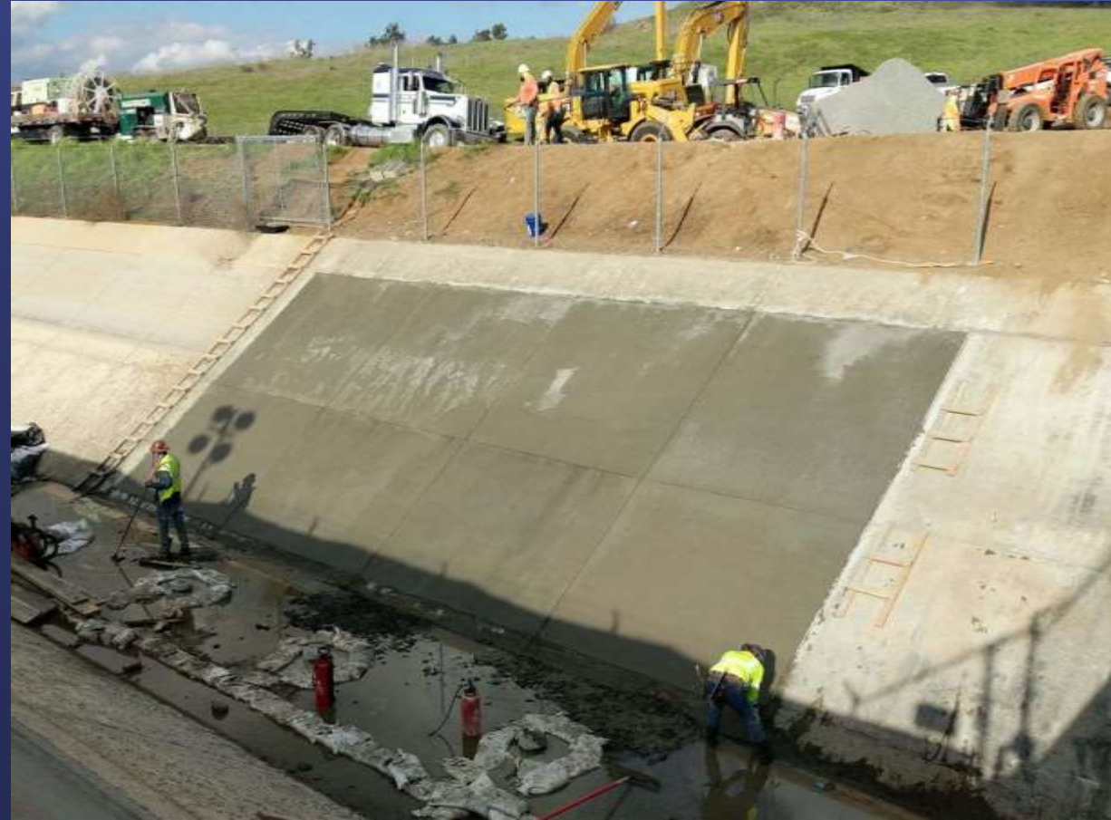
Concrete Panel Installation
