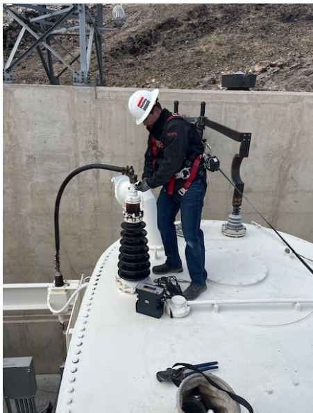
Staff testing the 230kV transformers at Eagle Mountain pumping plant
