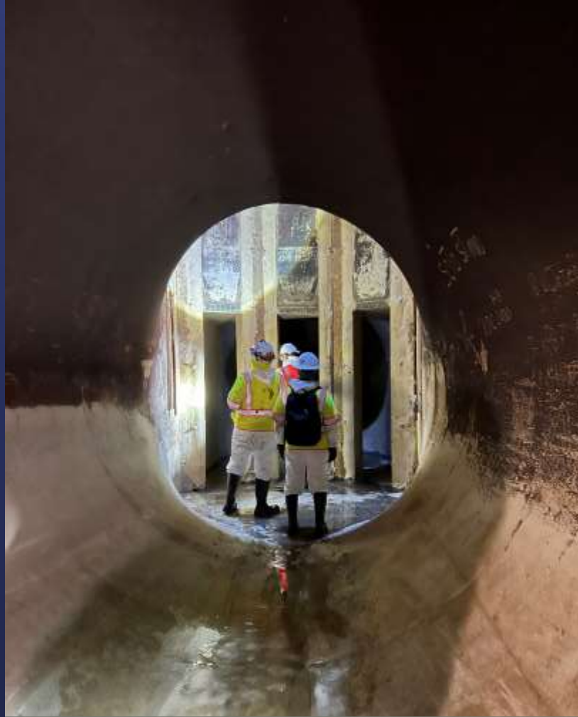
Inspection – San Gabriel Tower
