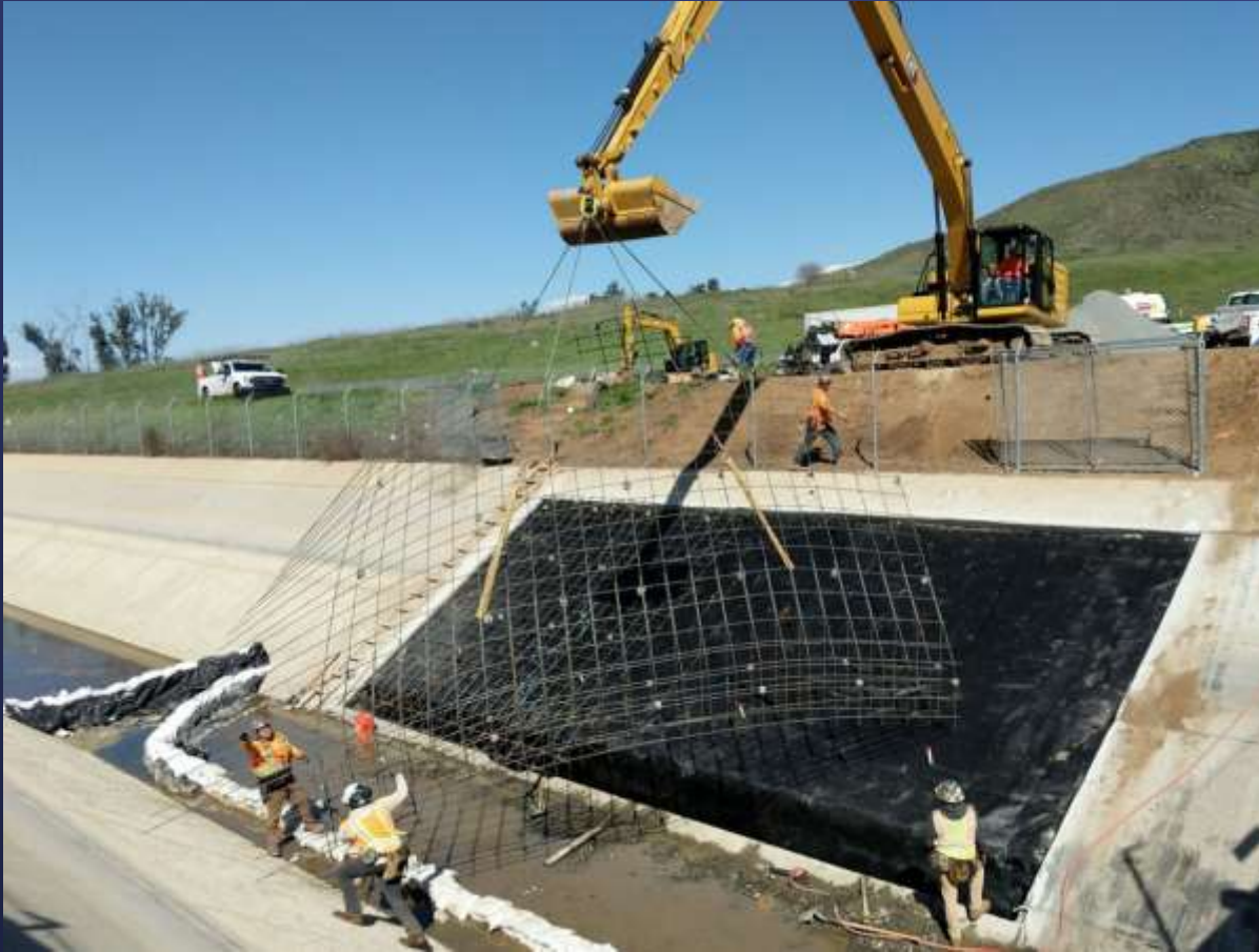
Reinforced Steel Installation
