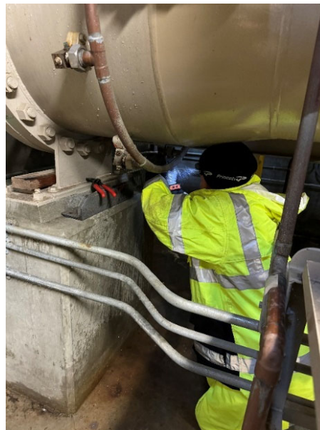
Staff performing venturi meter maintenance at the Skinner plant
