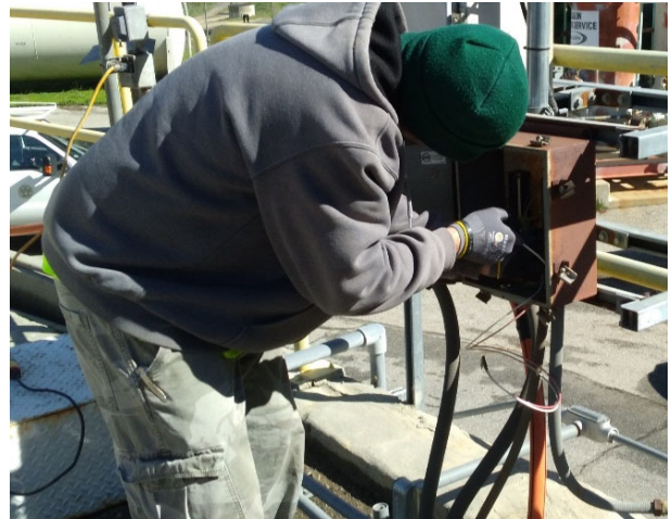
Staff installing electrical conduit at Magazine Canyon Junction Shaft
