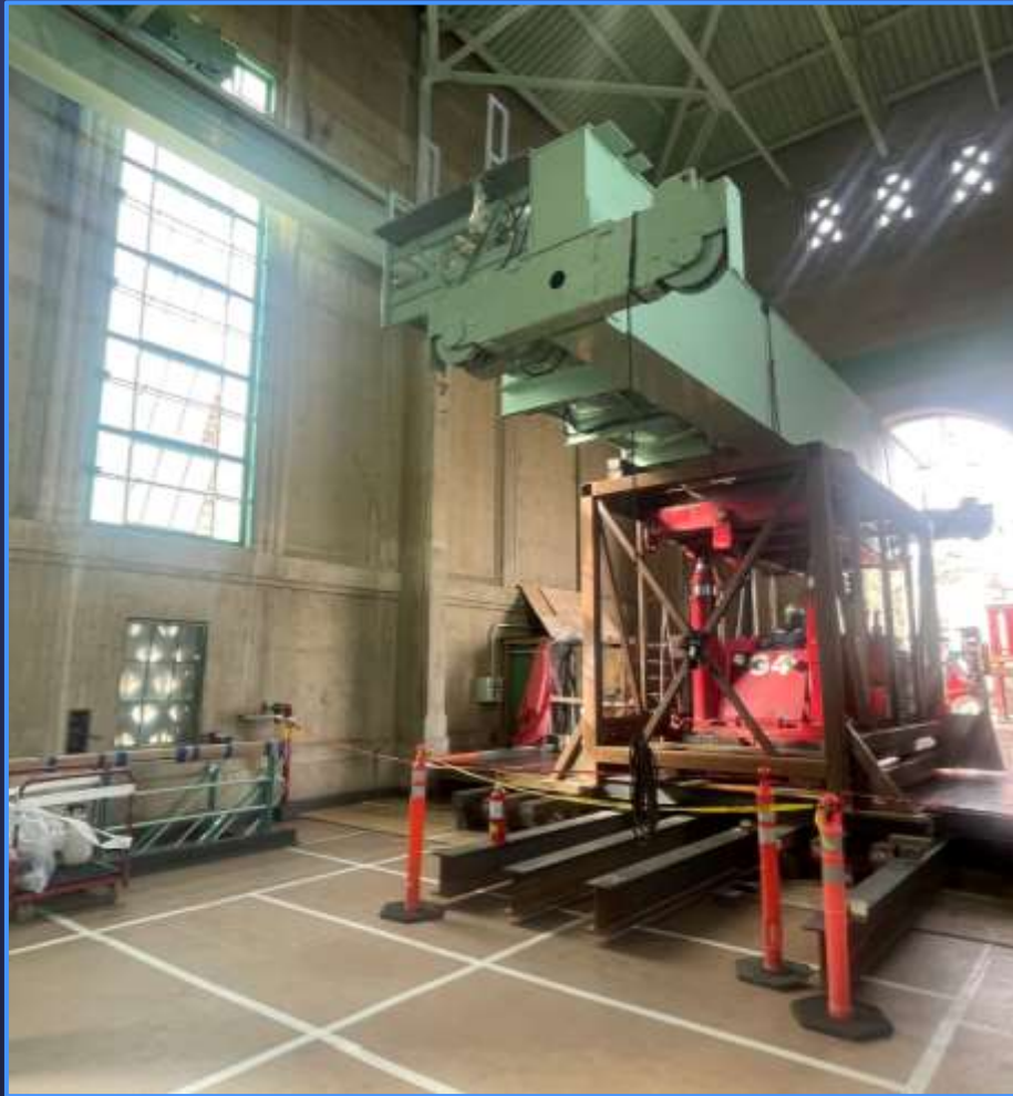
Installing the overhead crane girder at Eagle Mountain Pumping Plant
