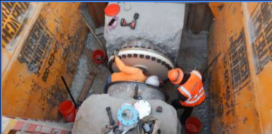
Bolt Up of 42-inch Blind Flange
