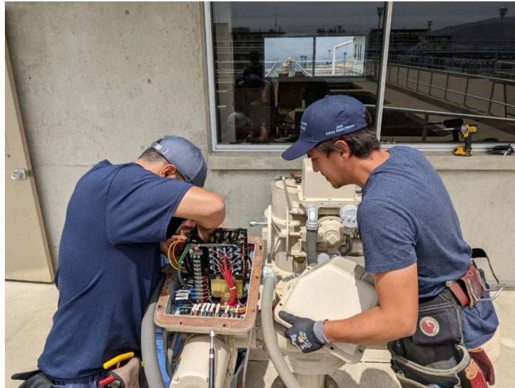
Staff upgrading filter valve actuator spring packs at Diemer plant
