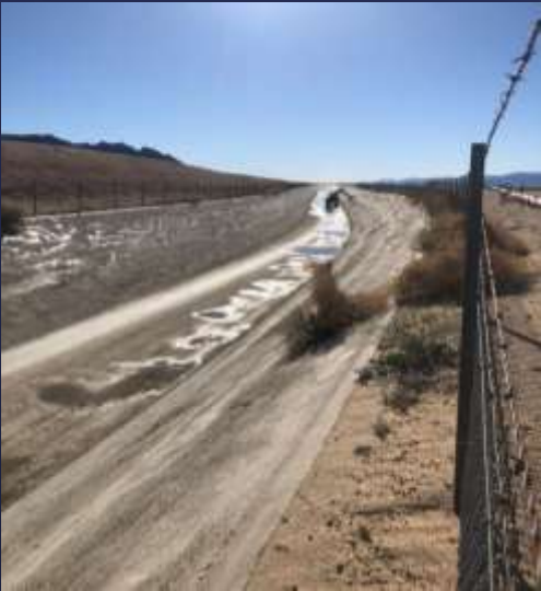
Colorado River Aqueduct
