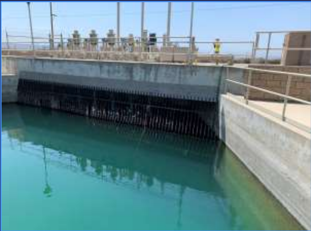
Bypass Channel Inlet
