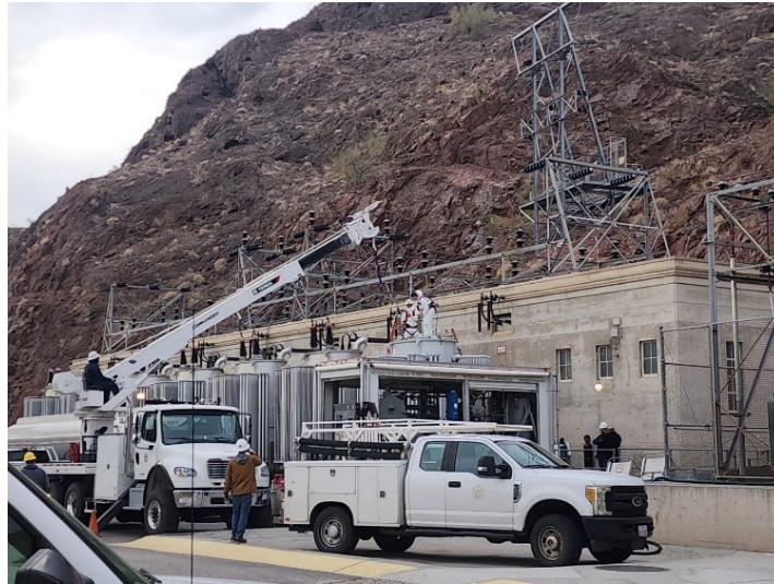
Staff replacing secondary bushings at Intake Bank transformer on the CRA
