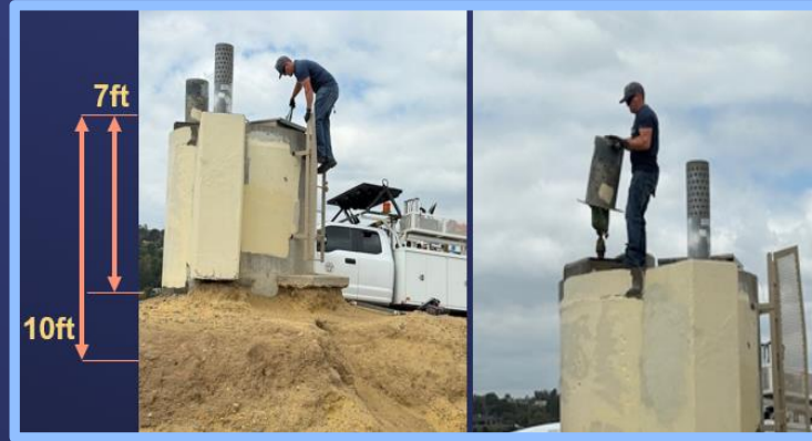
Install fall protection
