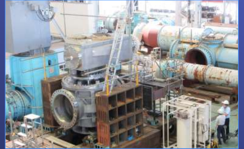
Fabrication of 48-inch Diameter Valve
