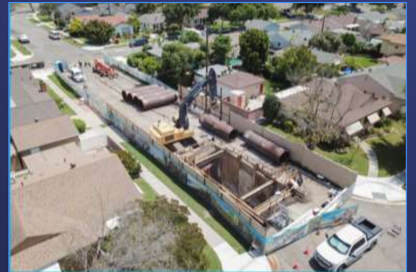
Typical Pipe Access and Storage Site
