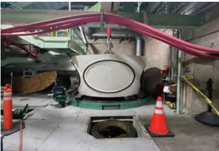
Discharge valve plug being installed after coating at Iron Mountain
