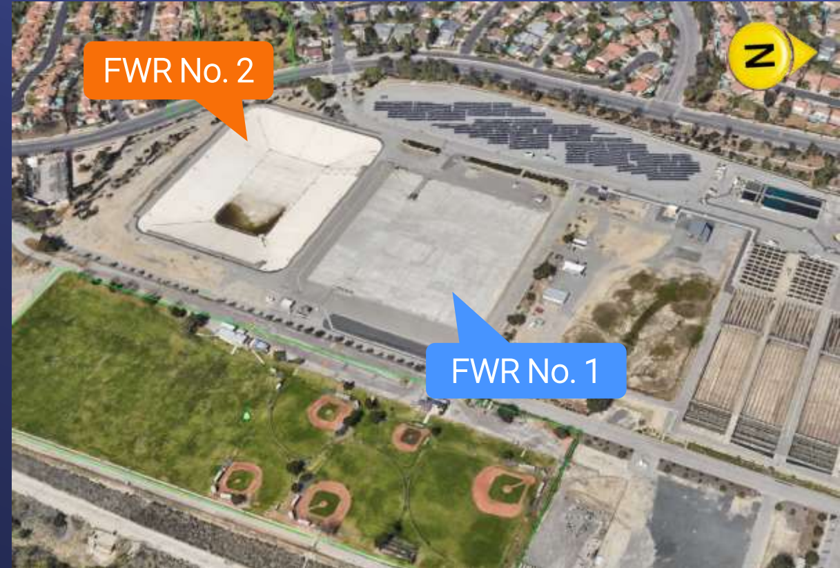
Joseph Jensen Water Treatment Plant
