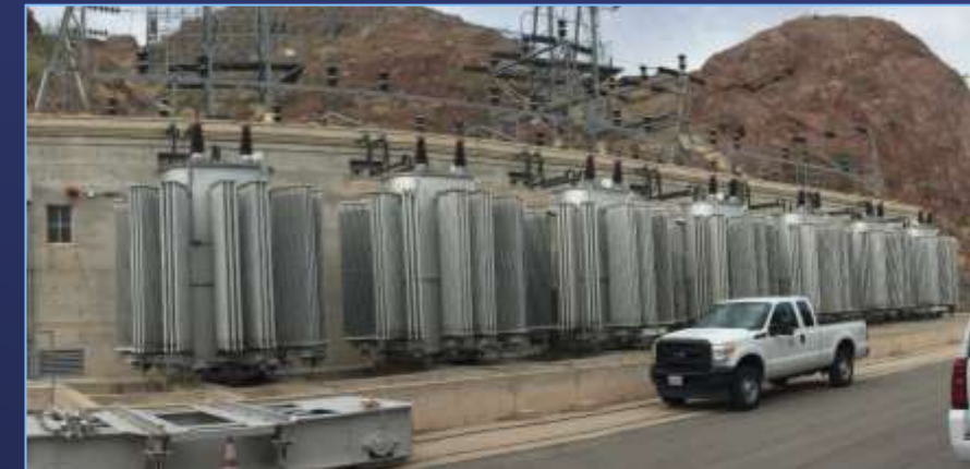
Intake Pumping Plant
