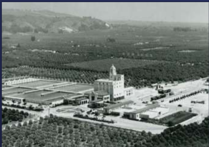
Softening and Filtration Plant, 1940s (Weymouth Plant)
