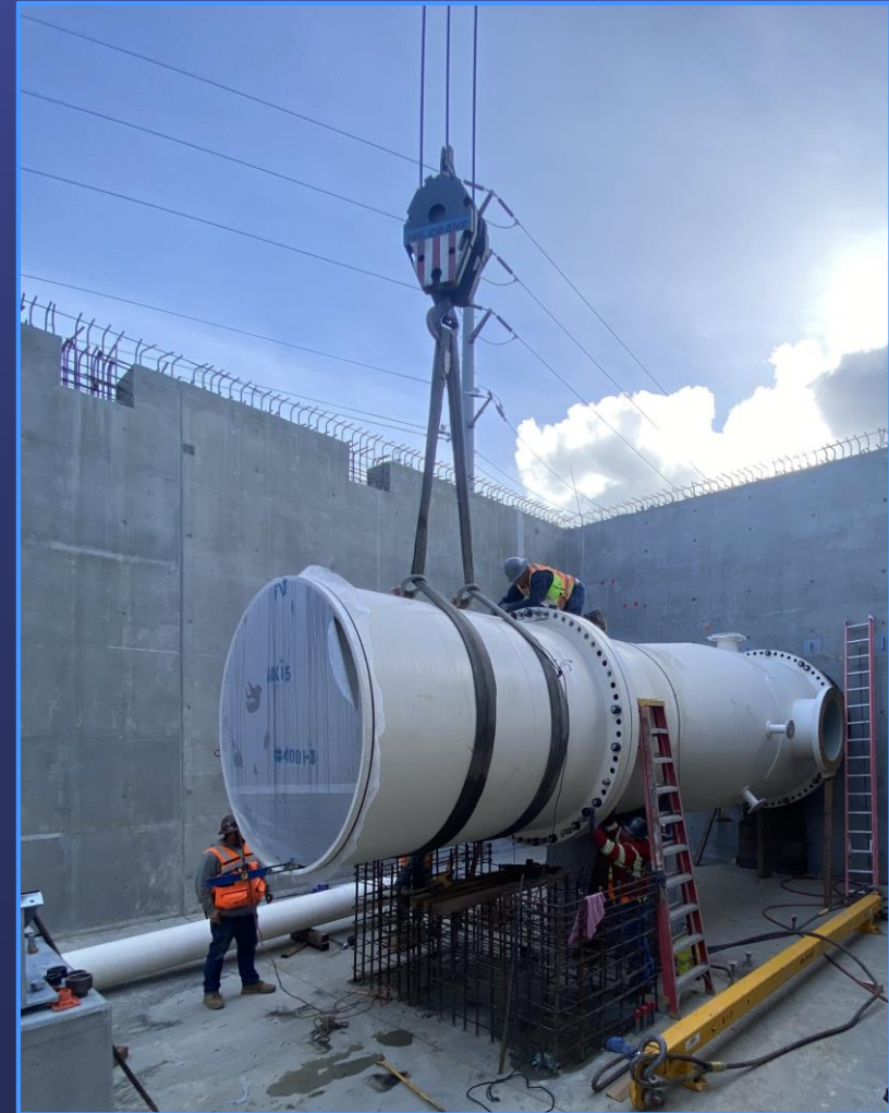
Placement of 96-inch bypass pipeline for Wadsworth Pumping Plant Bypass Pipeline
