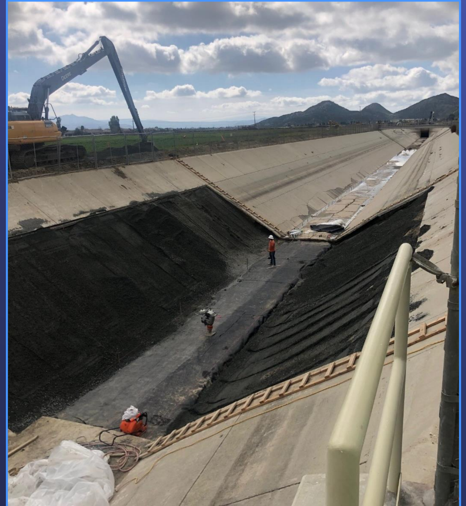
Contractor compacting aggregate base material along side slopes of San Diego Canal
