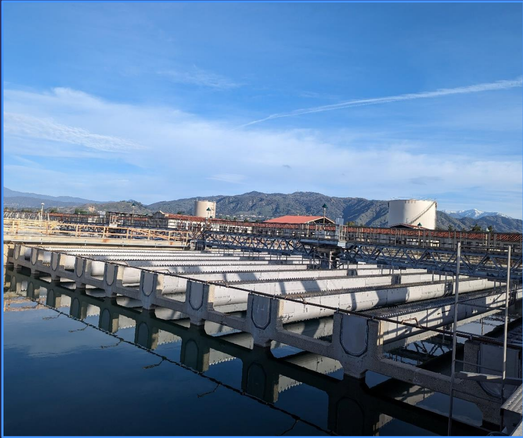
New stainless-steel launders in Basin 8
