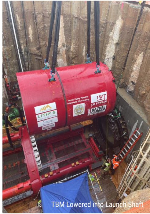
Tunnel Launch Shaft
