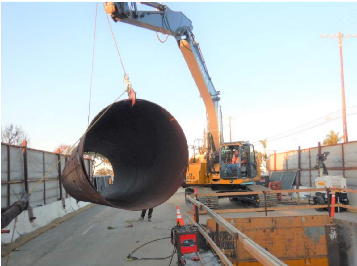
Second Lower Feeder Reach 3B— Contractor Installing Steel Liner in Portal
