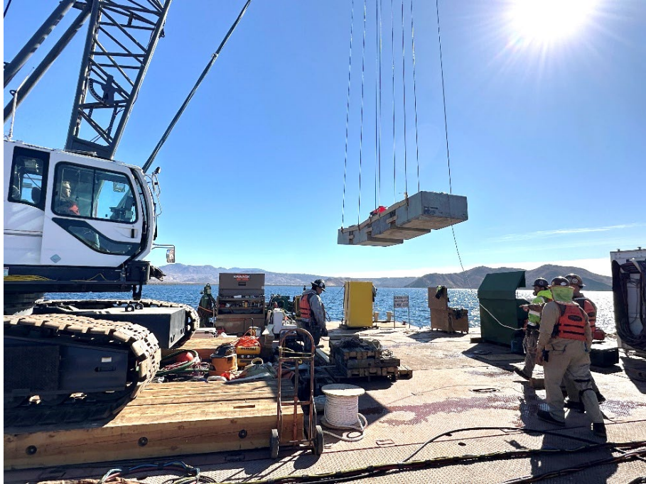
Diamond Valley Lake Wave Attenuator Replacement — Hoisting Anchor Blocks into Water
