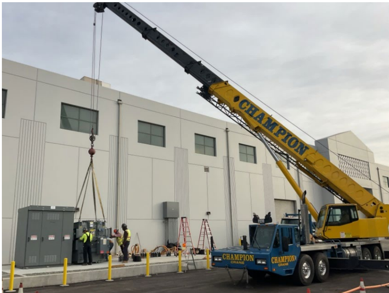
La Verne Shops Improvements – New Unit Substation Transformer Installation
