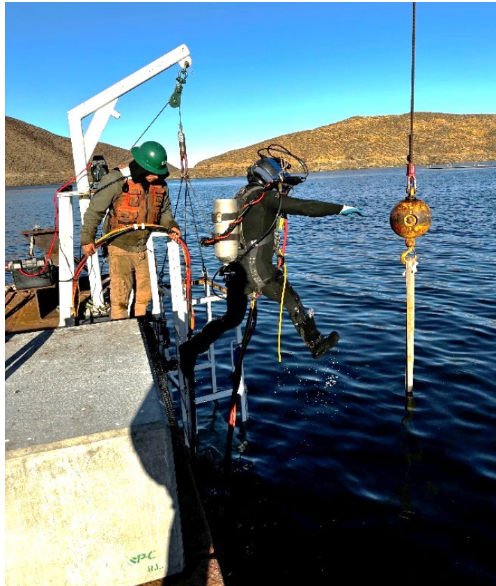
Diamond Valley Lake Wave Attenuator Replacement — Diver Entering Water for Block Installation
