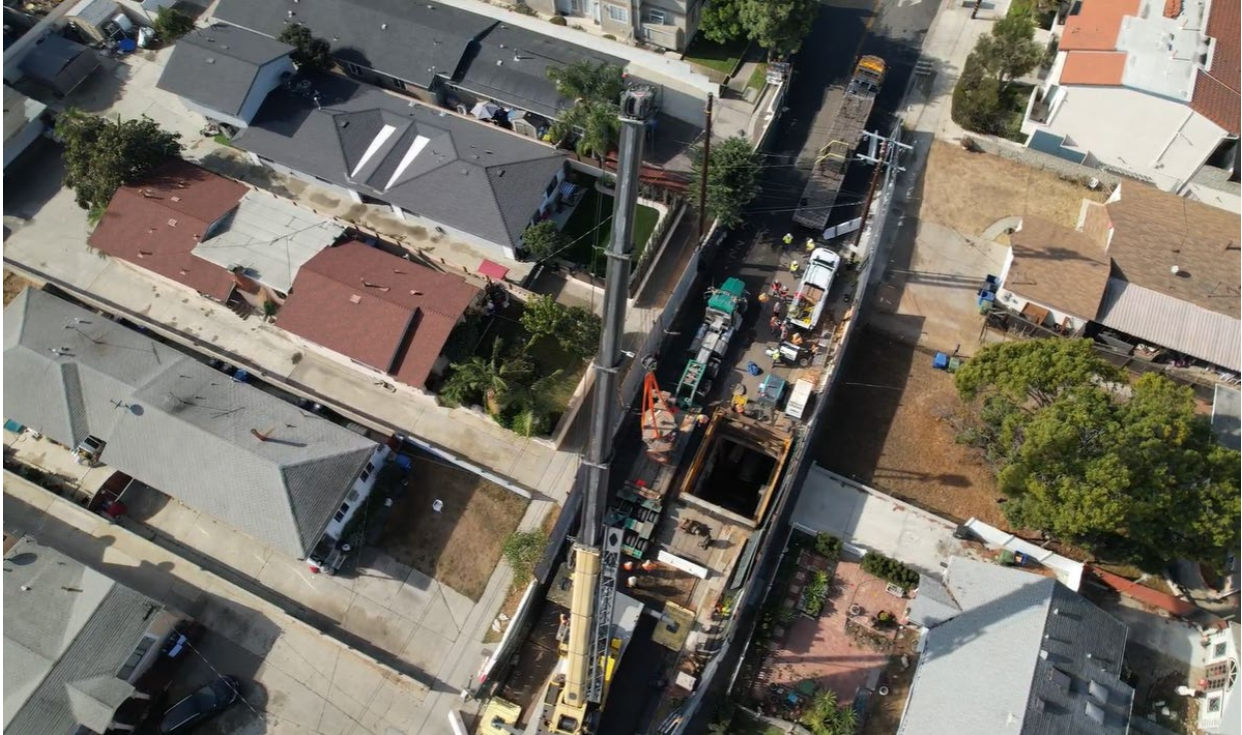
Second Lower Feeder Reach 3B— Removing Old Valve from Vault
