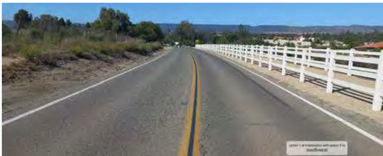
Photograph No. 4: Los Alamos Road BH-15, facing southwest.
