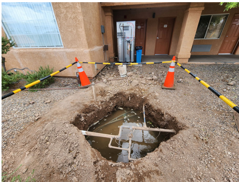
Plumbing staff repaired a leak in the fire water system.
