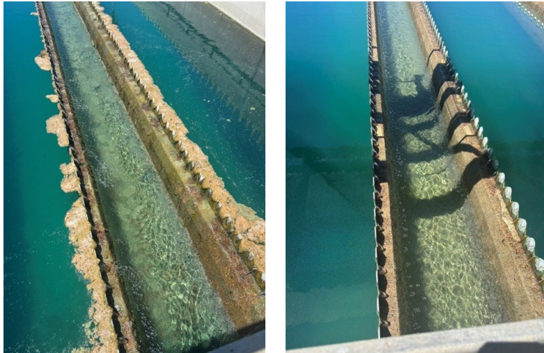
Module 3 Launder and Basin Cleaning
