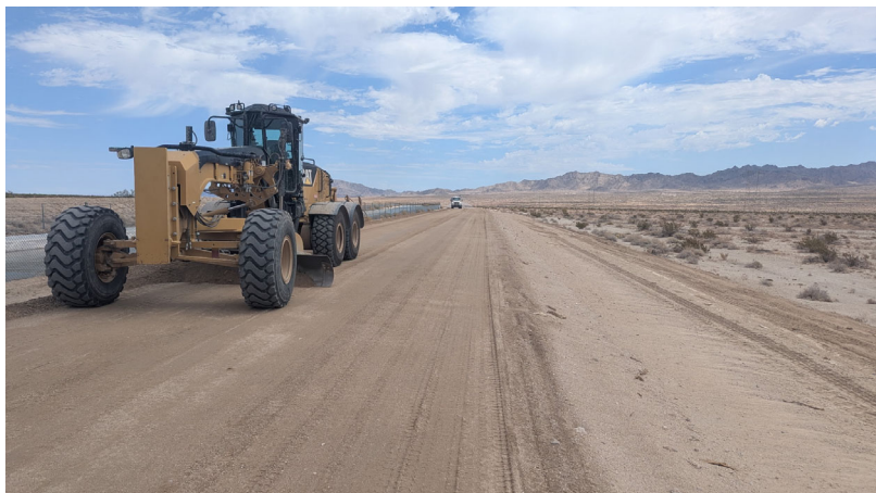
Staff performing storm damage repairs.
