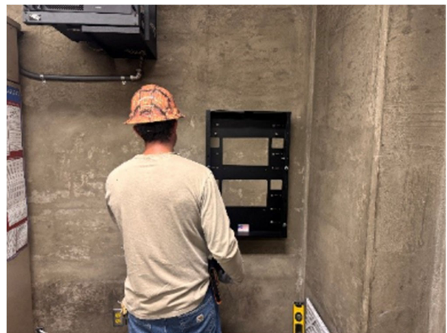
Staff installing conduit (left) and enclosure (right) for improved communication systems at Rio Hondo HEP.
