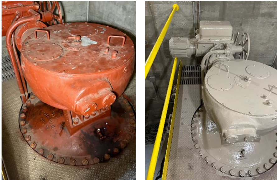
Before and after coating on a 30-inch valve.
