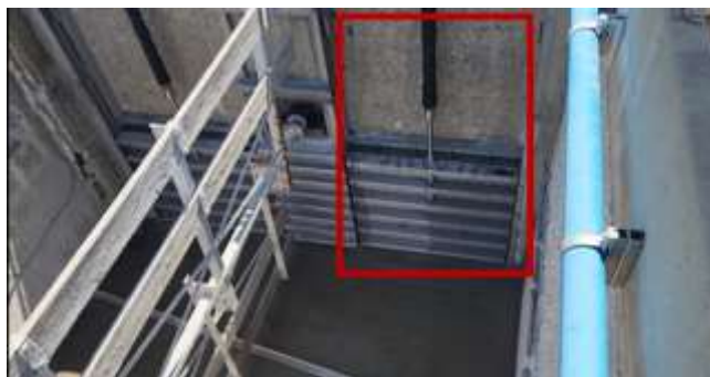
Weymouth basin influent slide gate in closed position
