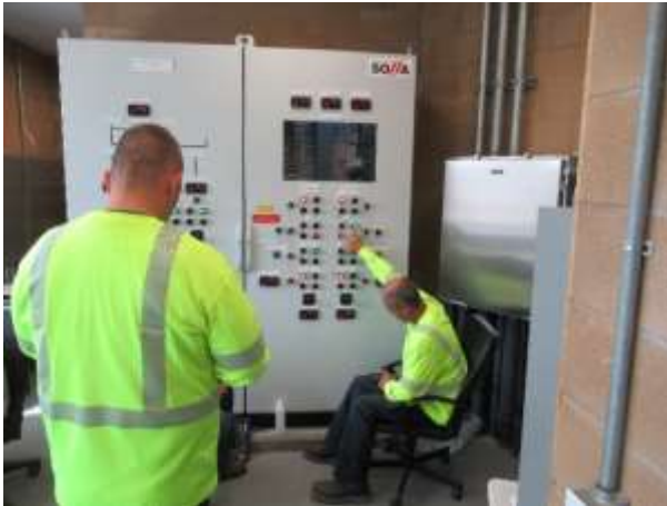
Staff operating a valve to begin the surge test (left) and monitoring the surge test (right) at Greg Avenue Pump Station
