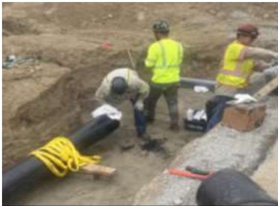
Staff installing a drain line (left) and taking delivery of ballast rock (right) for the heli-hydrant facility at Diemer plant
