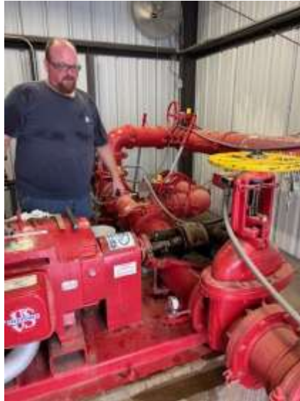
Staff rebuilding a fire pump at Gene pumping plant
