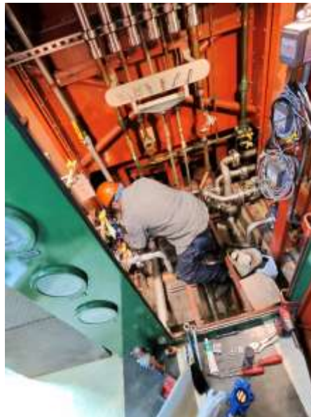
Staff installing new stainless steel plumbing on a CRA pump motor
