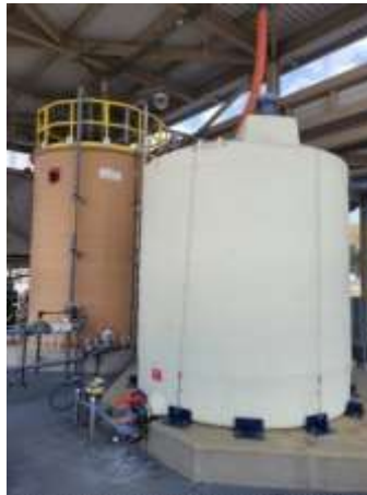
Temporary fluoride tank at the Jensen plant
