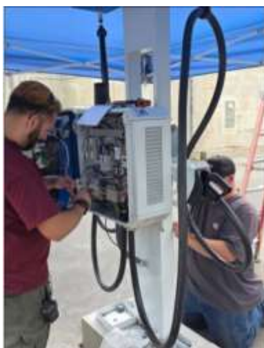
Staff installing a charger station (left) and two completed charging stations (right)
