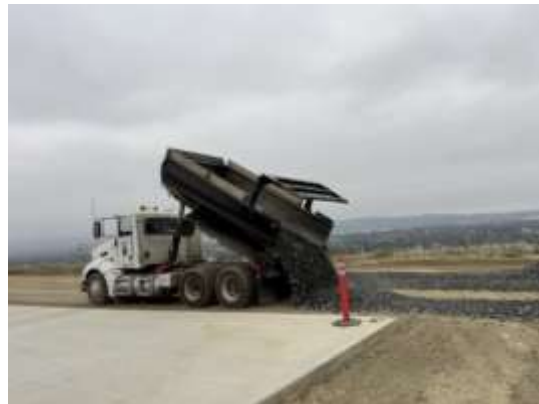
Staff installing a drain line (left) and taking delivery of ballast rock (right) for the heli-hydrant facility at Diemer plant
