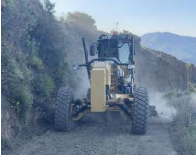
Staff performing routine grading at Pleasants Peak
