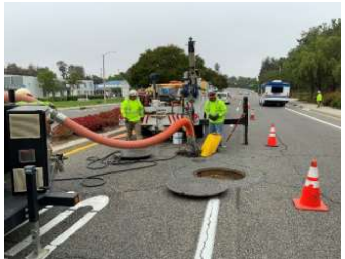
Staff setting up traffic control (left) and dewatering set-up during the San Diego Pipeline No. 4 shutdown (right)
