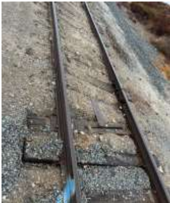
Damaged track (left), track during repairs (middle), and first railcar delivery after track repairs (right)
