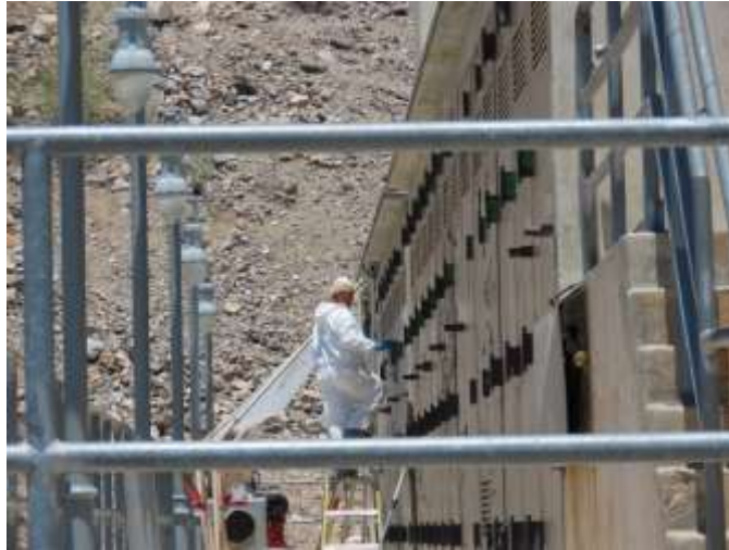
Staff preparing the surface of circuit breaker enclosure for new coatings at Hinds pumping plant
