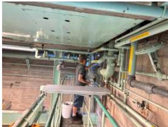
Staff installing wiring for a new lubrication system control valve at Gene pumping plant
