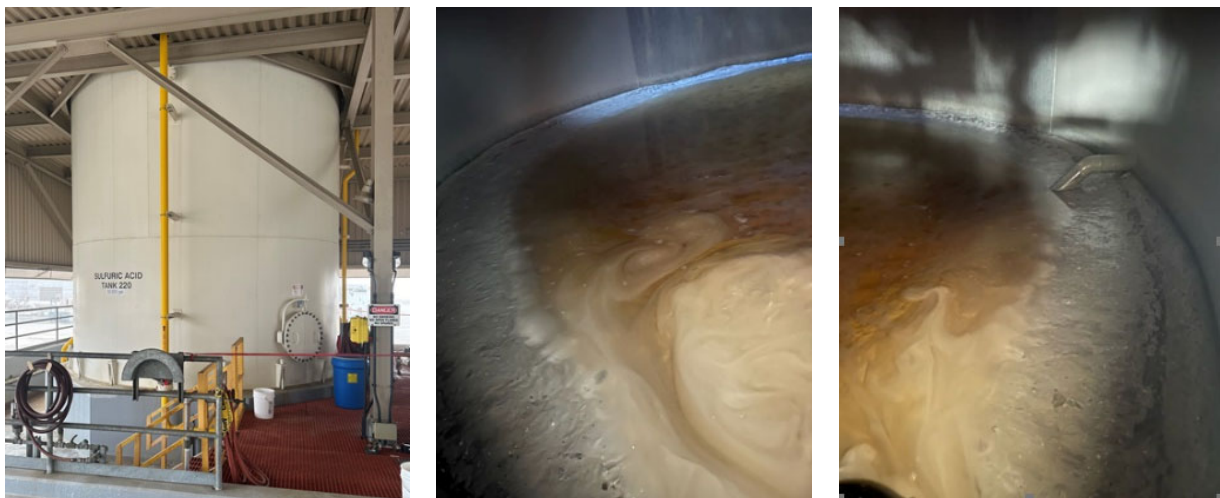
Sulfuric Acid tank and inside tank clean-out
