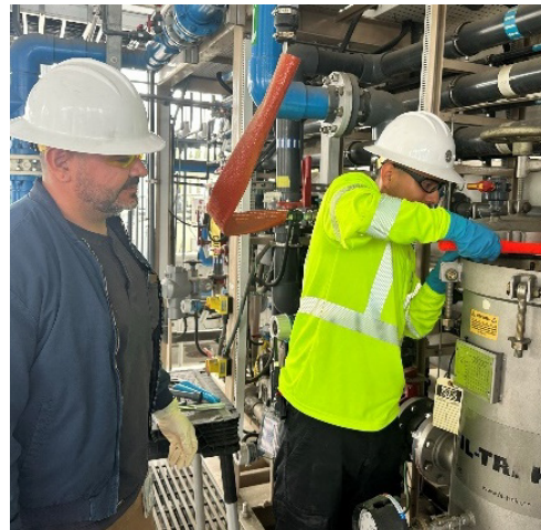
Preparing microbiological samples for analysis (left) and replacing cartridge filters (right) at the PWSC Napolitano Innovation Center
