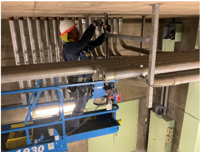
Staff installing new brackets and conduit for fiber optic cable at the Temescal HEP
