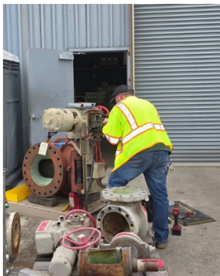
Staff setting valve limits (left) and rewiring and testing valves (right) at Covina PCS
