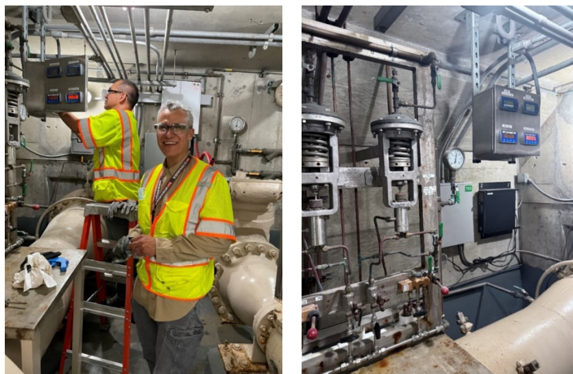
Staff installing valve position displays at Beverly Hills PCS
