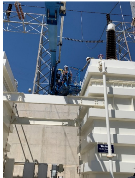
Staff connecting 230kV bus to Hinds spare transformer (left) and installing spare transformer neutral CT (right)
