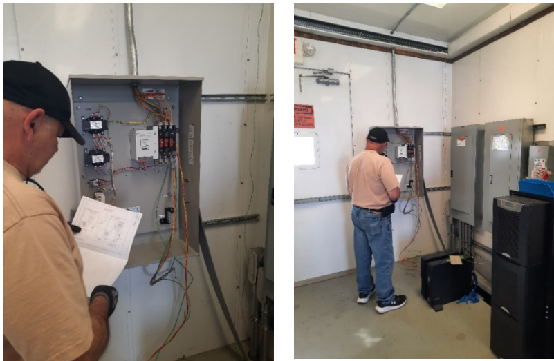
Staff installing an automatic transfer switch on a chemical feed system at the Diemer plant
