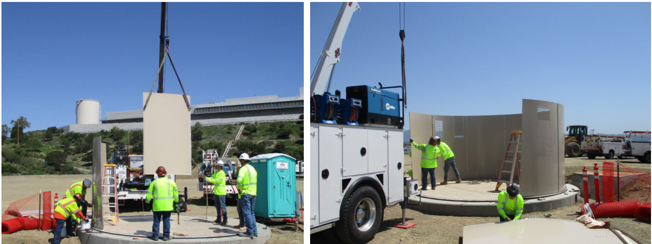
Staff erecting the helicopter hydrant water tank at the Diemer plant
