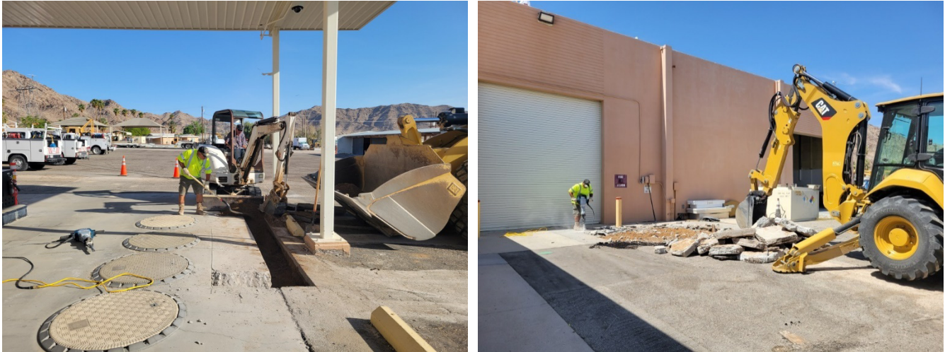
Staff installing a new conduit run for the Iron Mountain fuel island
