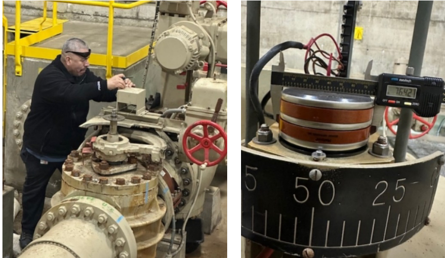
Staff measuring existing potentiometer (left) and potentiometer (right) at Covina PCS
