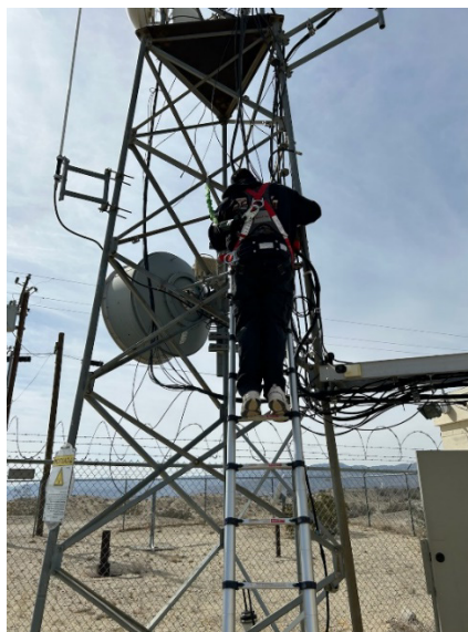
Staff installing new radios and antennas for CRA gauging stations
