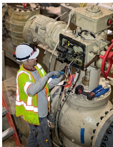
Staff setting valve limits (left) and rewiring and testing valves (right) at Covina PCS
