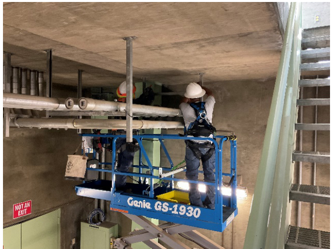
Staff installing new brackets and conduit for fiber optic cable at the Temescal HEP
