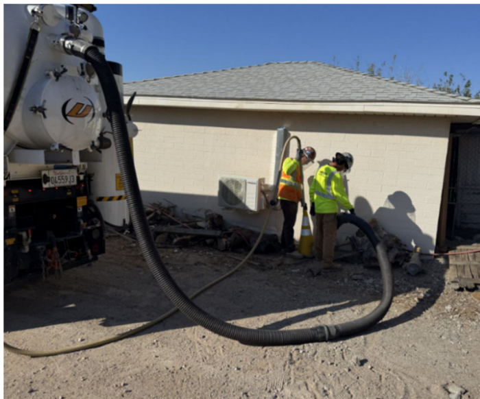
Staff potholing to inspect domestic water lines at Hinds pumping plant
