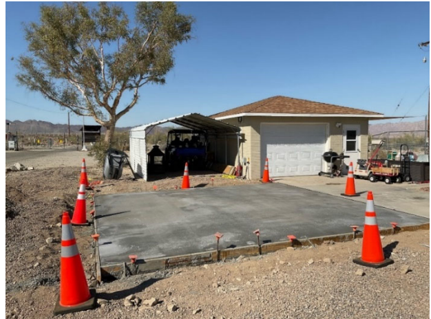
Grading preparation (left) and concrete placement for carport construction (right) at Eagle Mountain village
