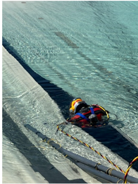
Initial dive to reinforce both sides of the floating cover tear at Garvey Reservoir
