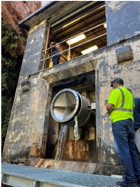
Testing of newly installed dam valve at Gene Wash Reservoir
