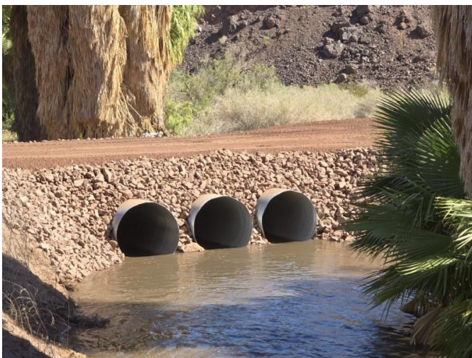
New 42-inch culverts and final grading
