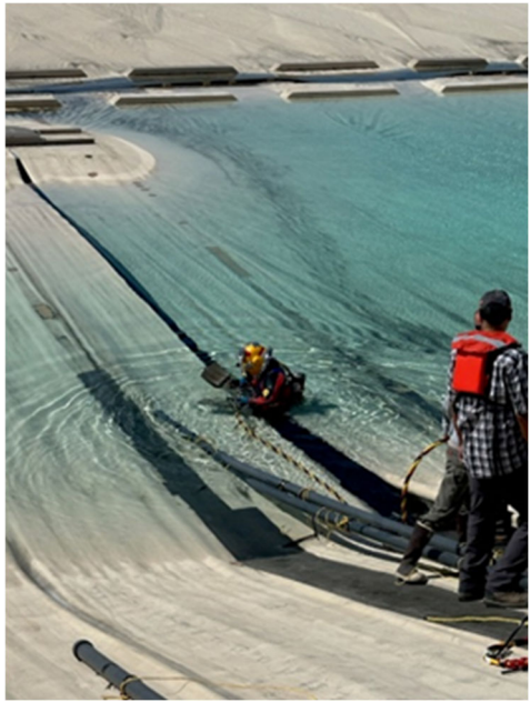
Initial dive to reinforce both sides of the floating cover tear at Garvey Reservoir
