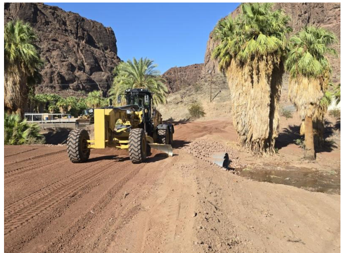
New 42-inch culverts and final grading
