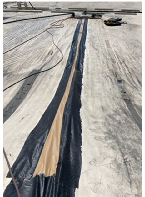
Staff pulling tear together (left), patching tear (middle), and completed repair (right)
