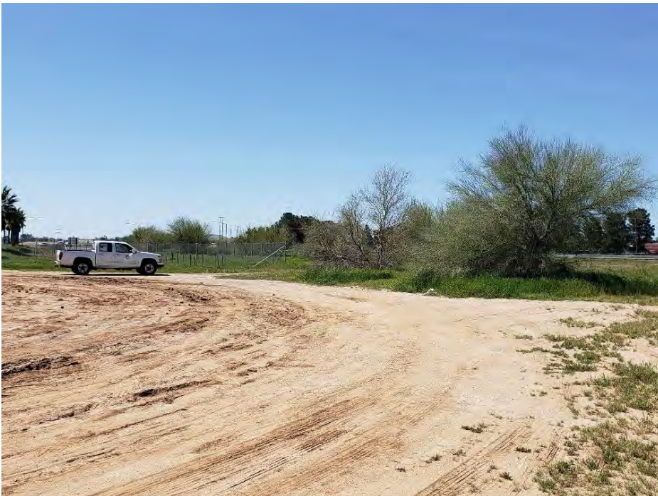
Photograph 4. Along Van Buren Boulevard just east of I-215, and across from March Air Reserve Base museum, facing south. Construction activities at this location include temporary treatment plant 2 and access. "Depression" is located behind the parked white truck inside the fence.
