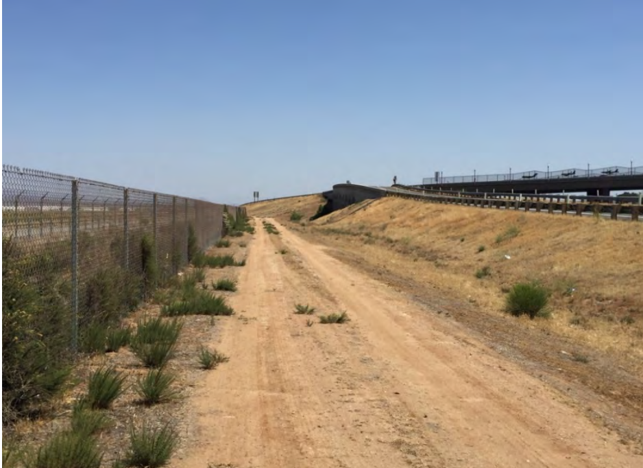
Photograph 3. Dirt access road between March Air Reserve Base and Van Buren Boulevard/I-215 overpass, facing south. Discharge piping would be constructed at-grade in this location.
