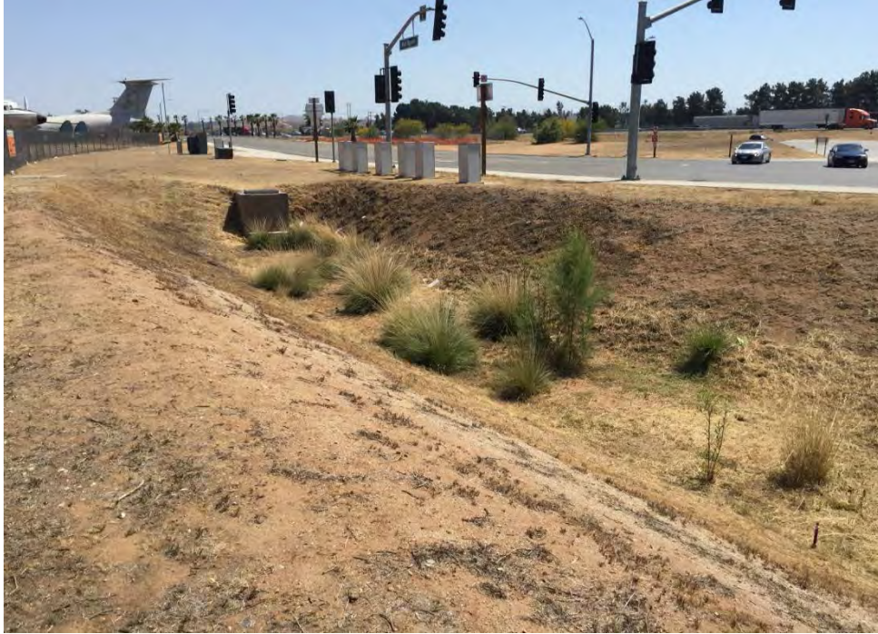
Photograph 1. Existing earthen dirt storm channel along Van Buren Boulevard just east of I-215 and north of the March Air Reserve Base, facing southwest.
