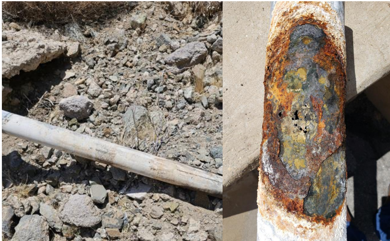
Existing asbestos cement pipe (left) and corrosion damaged pipe (right) at the Eagle Mountain Pumping Plant
