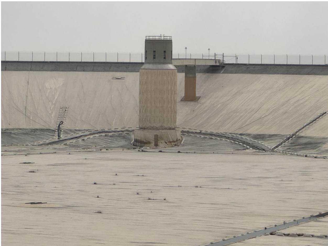
The existing reservoir floating cover and outlet tower at Garvey Reservoir
