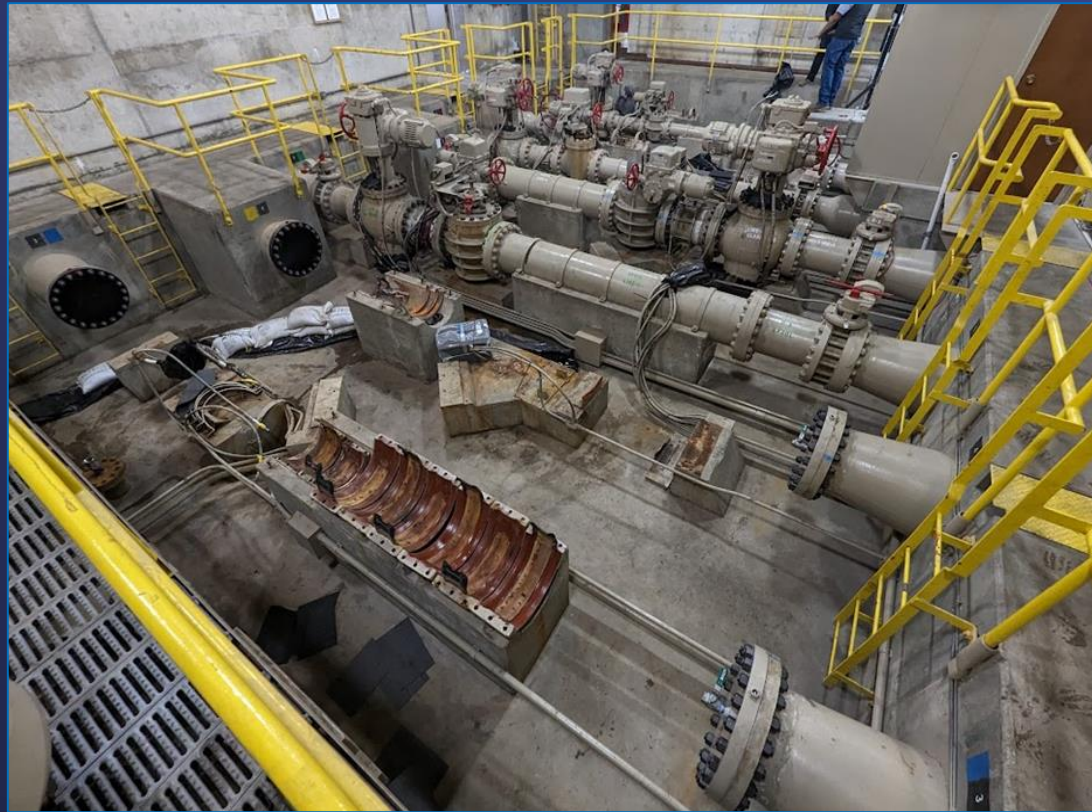
Covina Pressure Control Structure - Valve Replacement
