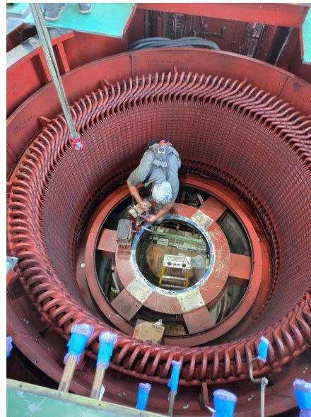
Removing the rotor and hydraulic jacks from Eagle Mountain Unit 9 stator
