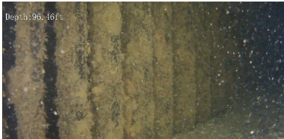
Inspection of valve inlet trash rack
