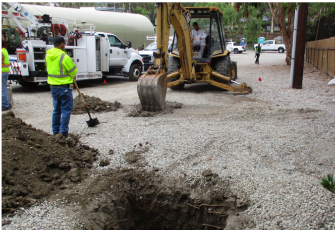
Excavating for percolation test pit (left) and conducting percolation test (right)
