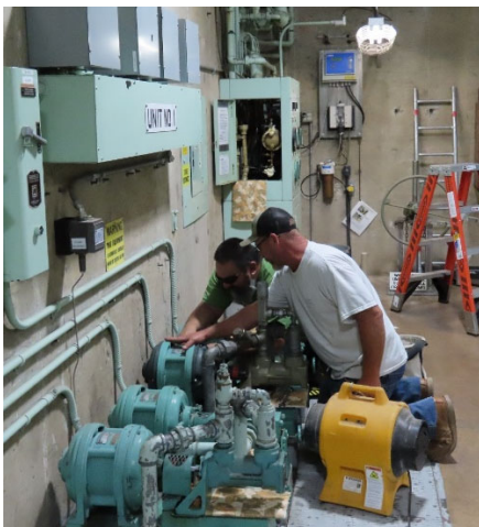
Removing a lubrication pump and motor for rebuild (left), splitter welding to build up worn areas (middle), and splitter weld repairs completed and ready for coating repairs (right)
