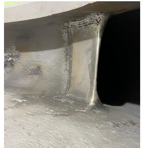
Removing a lubrication pump and motor for rebuild (left), splitter welding to build up worn areas (middle), and splitter weld repairs completed and ready for coating repairs (right)
