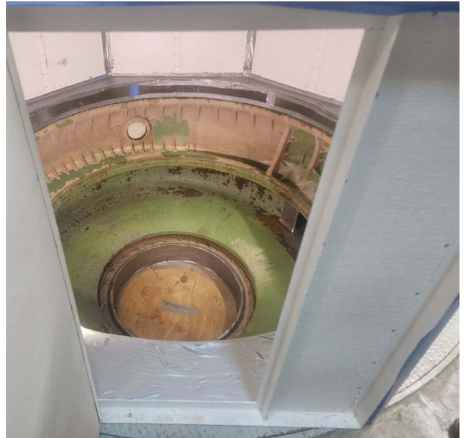
Installing pump bowl containment at Eagle Unit 9 (left), and a look inside the containment (right)
