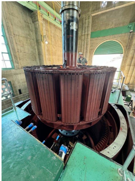
Removing the rotor and hydraulic jacks from Eagle Mountain Unit 9 stator
