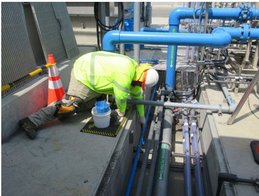
Staff coating pipes at Napolitano Center
