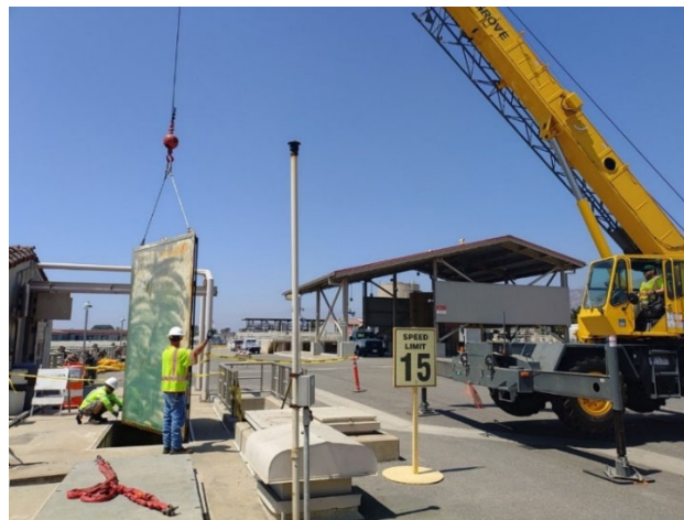
Mechanics removing filter effluent channel drop gate at the Weymouth plant
