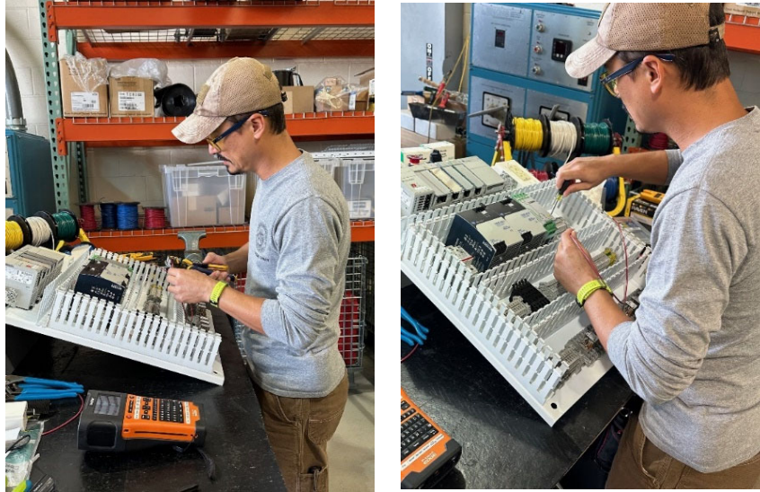
Staff is working on a nitrification control chemical feed system
