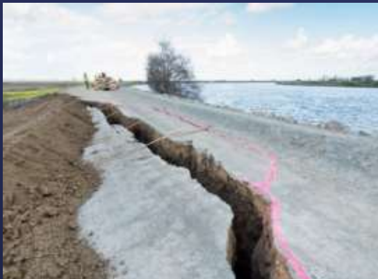
Levee Failure
