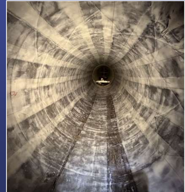
SDCWA's Carbon Fiber Lining Inspection
