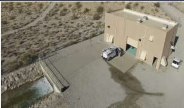
Desert Water Agency Hydroelectric Plant
