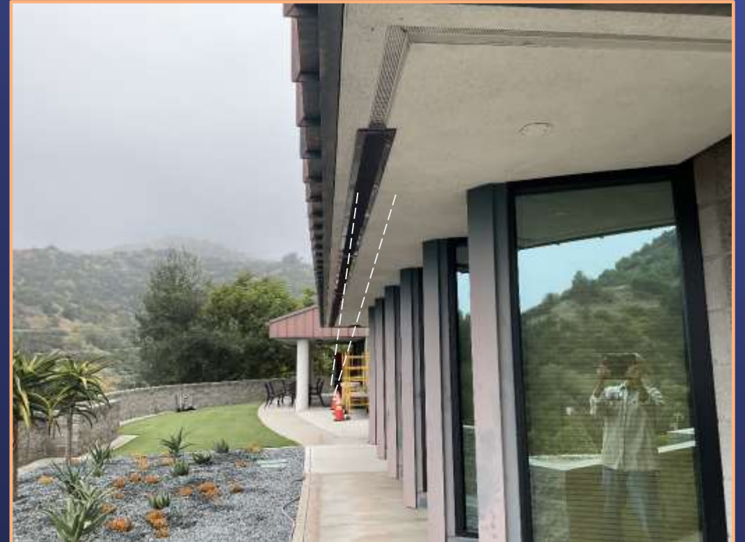
Main Building (Rear)
