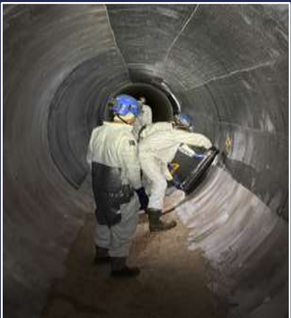
SDCWA's San Diego Pipeline 4 Repairs
