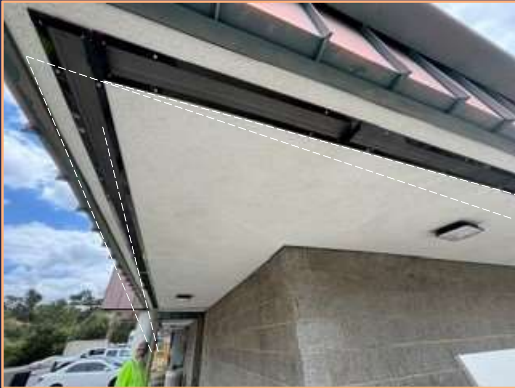
Main Building (Front)
