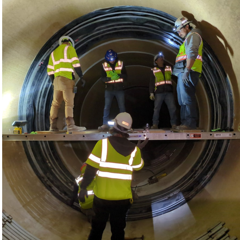
CRA Freda Siphon Seals Installation — Contractor Adjusting Retention Bands on the Seal
