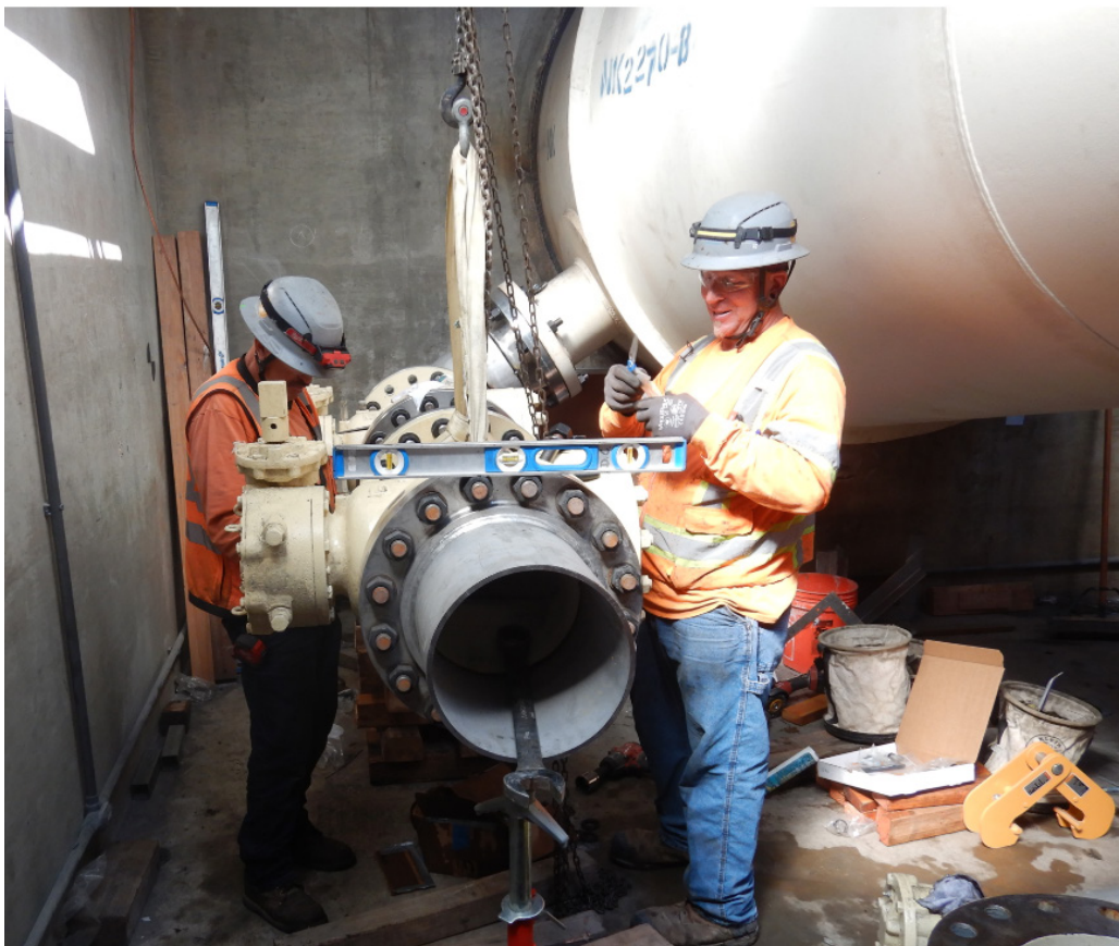
Second Lower Feeder PCCP Rehabilitation Reach 3B — Contractor Installing 12-Inch Bypass Piping
