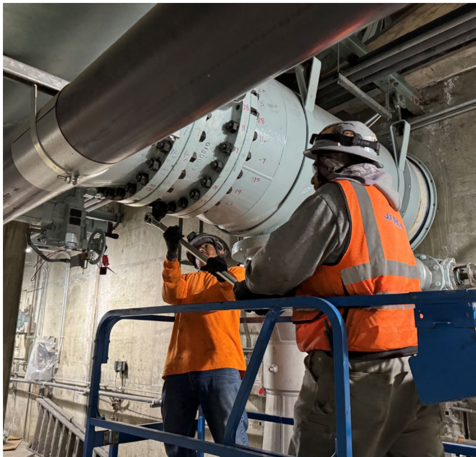
Weymouth Basins 5–8 and Filter Building No. 2 Rehabilitation — Torquing upgraded backwash valves at Filter 44
