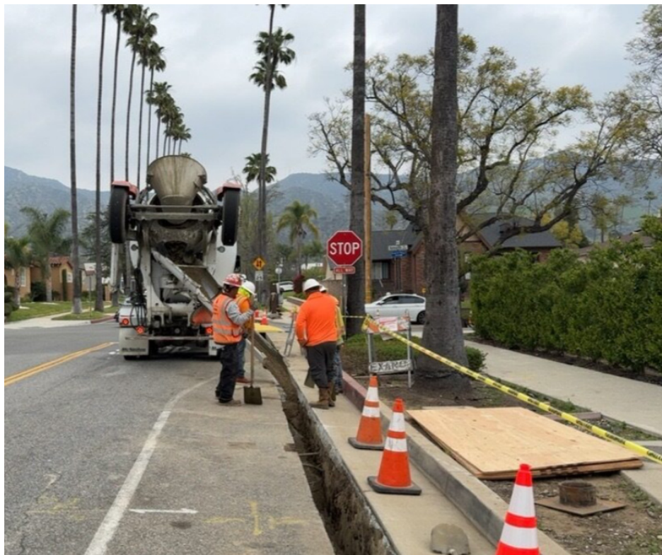
Santa Monica Feeder Cathodic Protection — Contractor Performing Slurry Backfill of the Anode Cables
