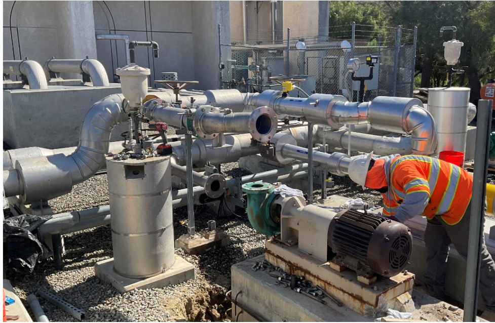
Service Connection OC -88 Chillers Replacement — Contractor Installing New Chilled Water Pump
